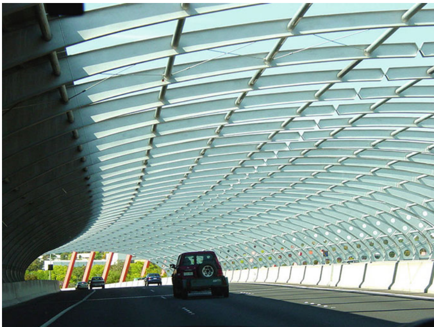
Fig. 1 Acoustic barriers on the Tullamarine Freeway, Melbourne, Australia [ photograph Atlantica , used under license (CC-BY-SA 3.0)]. For some burdens such as noise, there are engineering solutions available assuming sufficient mitigation costs are included in the initial project appraisal. Others such as the impact of automobile emissions and the particulate matter they produce on air quality may require policy action to limit certain vehicles and to encourage modal shift to less polluting forms of transport
