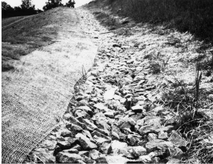
FIGURE 16.5 Rock channel lining.
