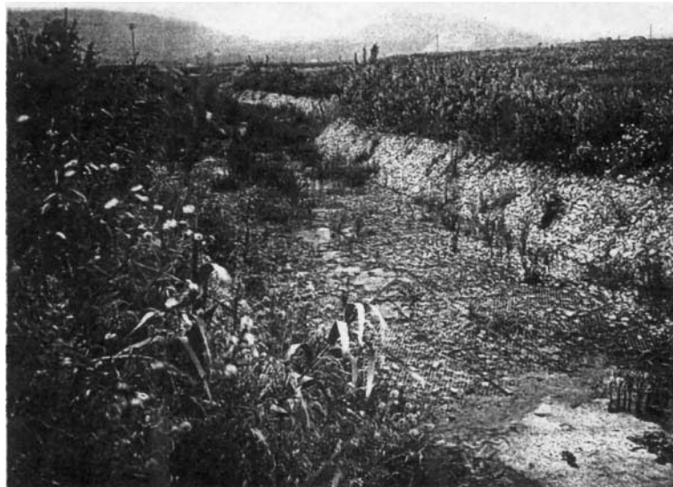
FIGURE 16.6 Wire-enclosed stone channel lining.
