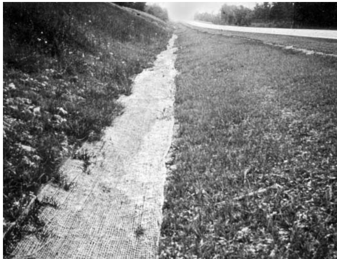
FIGURE 16.10 Jute net channel lining.
