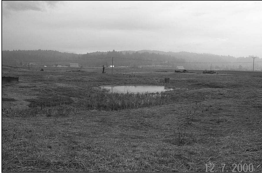
FIGURE 10.4 This stormwater treatment wetland was designed within an existing swale. Appropriate wetland vegetation was established at varying elevations above the dry-weather pool to provide treatment, soil stabilization, and aesthetics to the overall treatment wetland complex. Note this stormwater wetland does not discharge until the water surface elevation reaches the outlet works that is located at the upper right side of the impoundment area shown in this photograph. (Photograph by HWR, Inc. Arcata, California)
