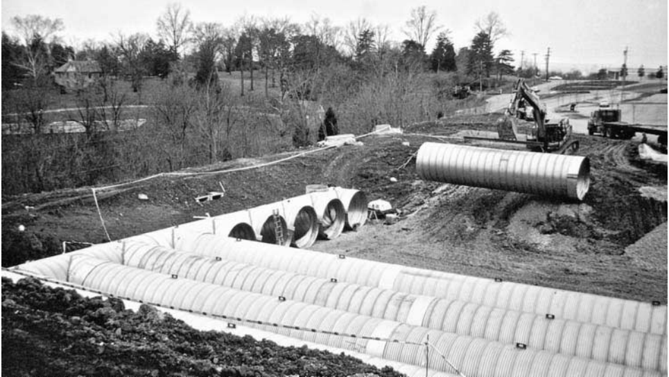
FIGURE 13.1 108" diameter detention system.
