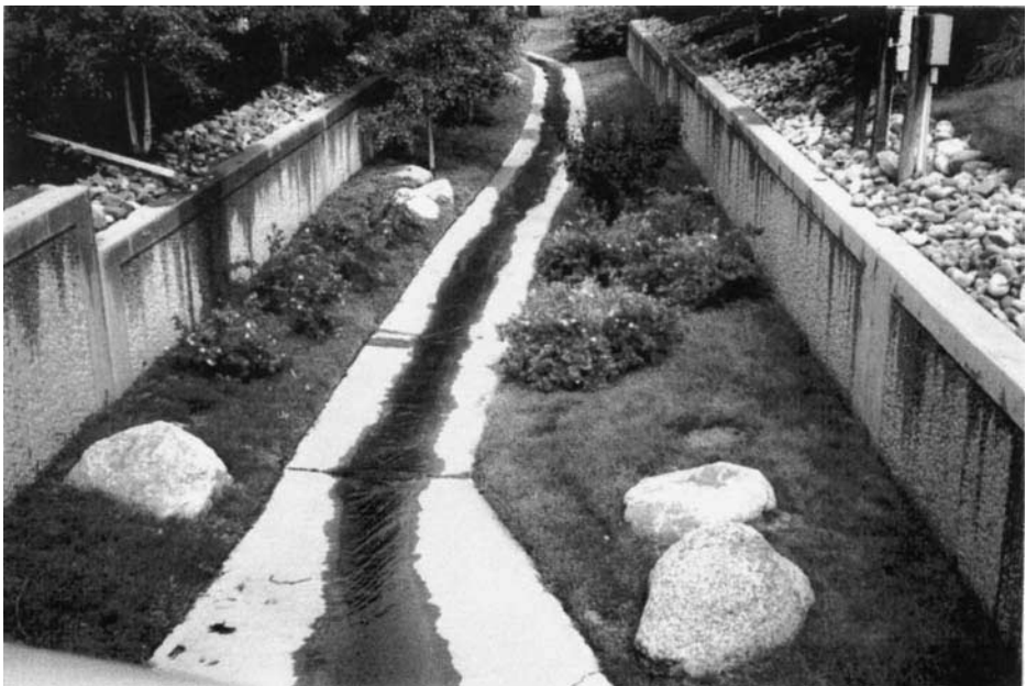
FIGURE 8.4 Example of channel detention by backwater depth.
