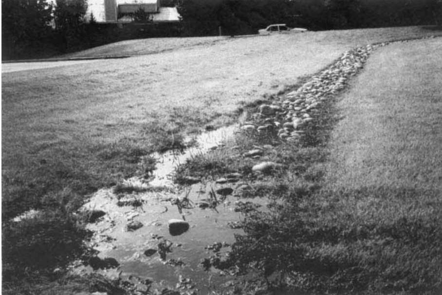
FIGURE 9.8 Standing water in infiltration basin as a result of clogging.
