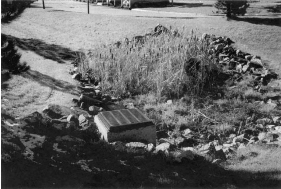
FIGURE 9.6 Small infiltration basin to catch stormwater from parking area.
