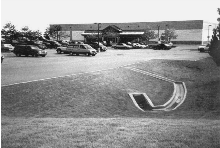
FIGURE 8.5 Detention system in parking area.
