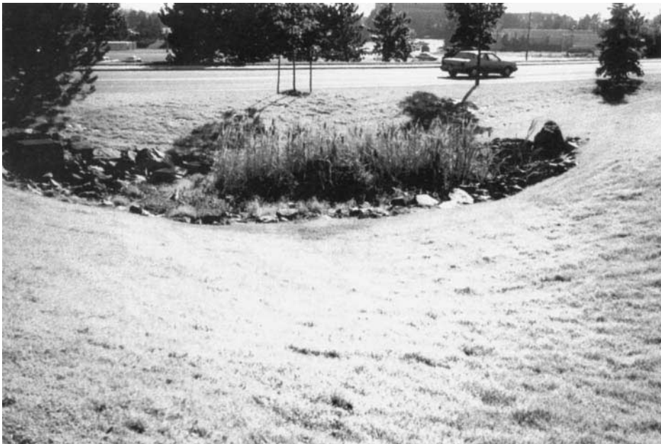
FIGURE 8.6 Infiltration and retention system.
