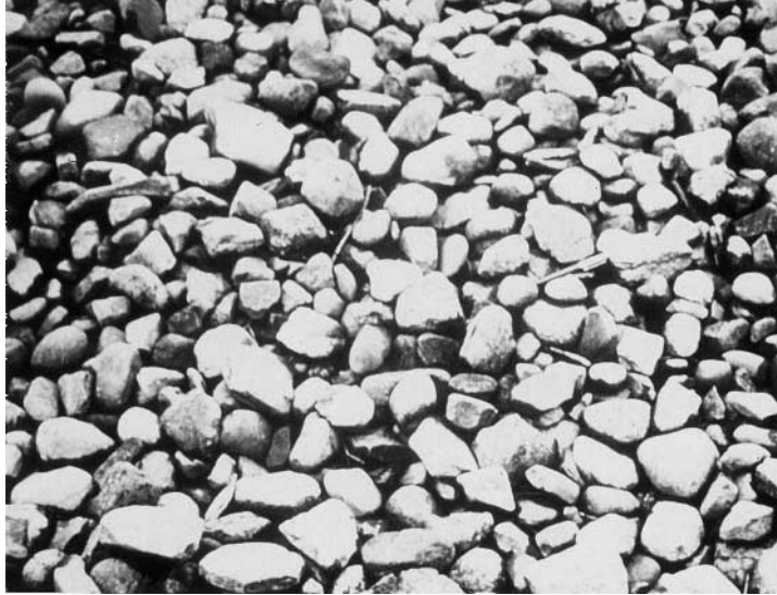
FIGURE 16.7 Gravel channel lining.
