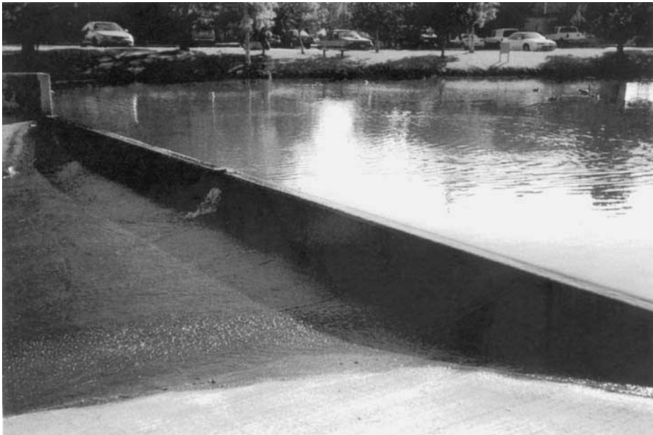
FIGURE 8.28 Spillway for a regional detention basin, Denver, Colorado.
