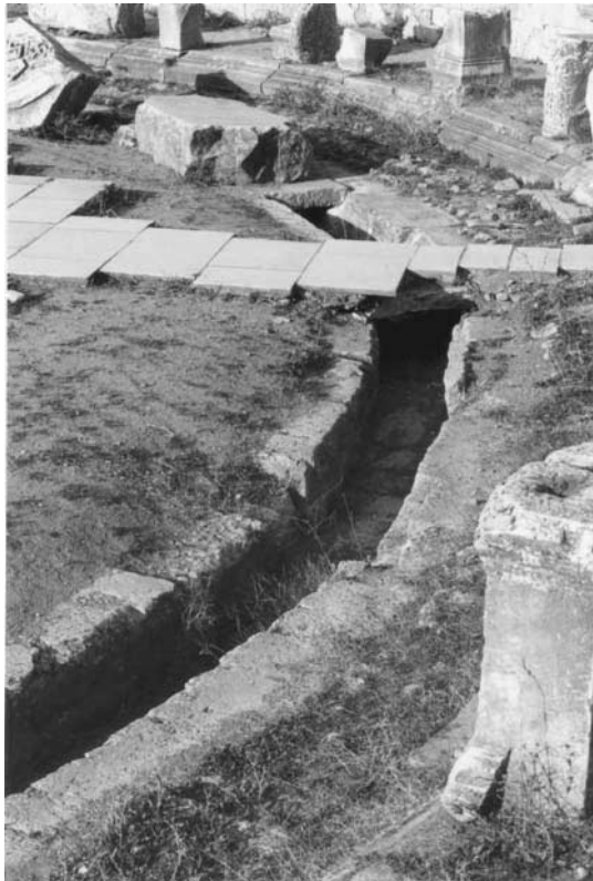
FIGURE 1.7 Drainage channel on floor of the Greek Theater at Ephesus. (Photo by L. W. Mays)
