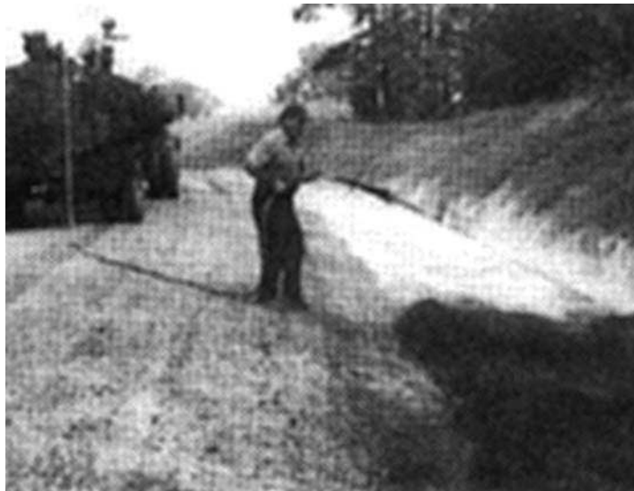
FIGURE 16.13 Fiberglass roving channel lining.
