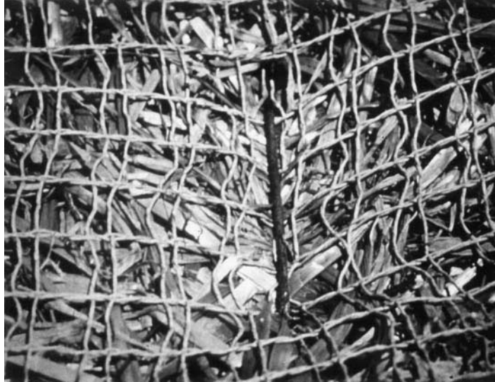
FIGURE 16.12 Straw with net channel lining.
