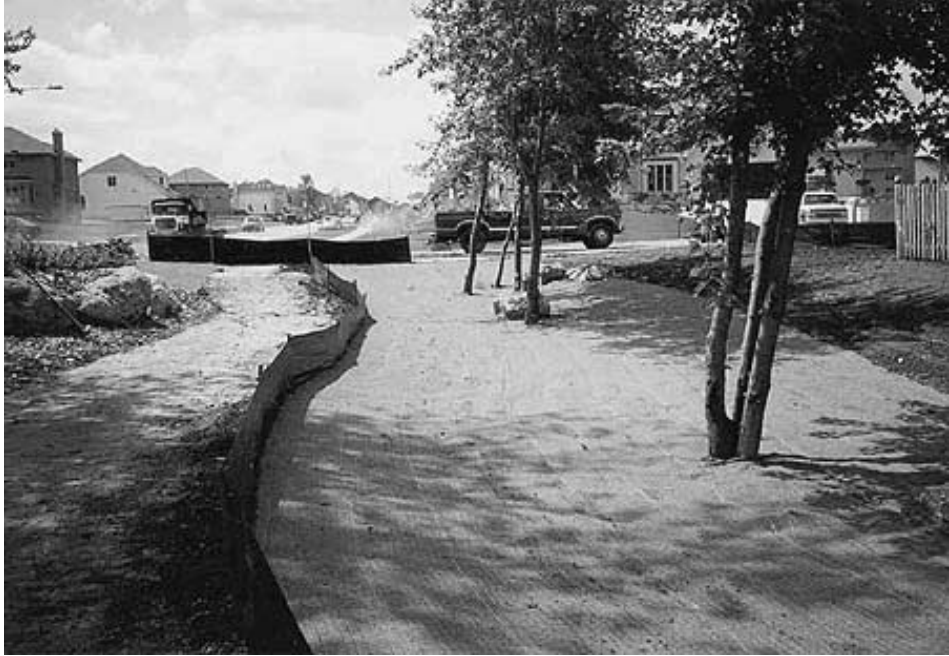
FIGURE 17.6 A channel that has been stabilized with TRM. (From IECA, 1998)
