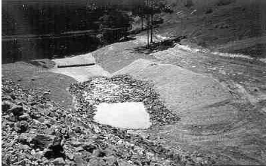
FIGURE 17.7 Riprap application. (From IECA, 1998)
