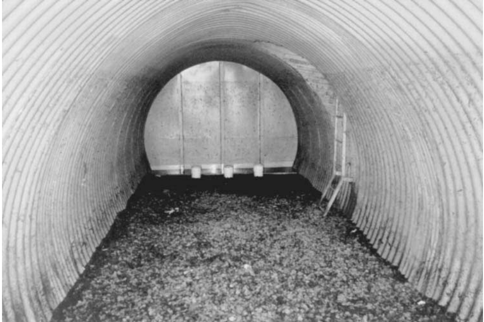
FIGURE 13.4 120" CSP sand filter.
