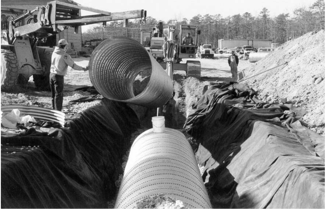
FIGURE 13.2 60" perforated CSP infiltration system.
