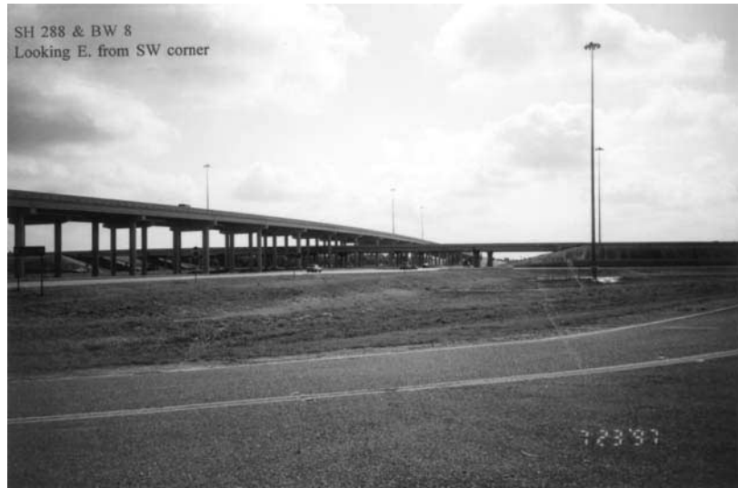
FIGURE 1.26 Detention pond at highway intersection of Beltway 8 and State Highway 288 South of Houston, Texas. (Photo by L. W. Mays)
