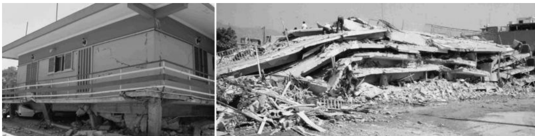
Figure 2.11 Typical collapses of frame buildings with open ground storey; ‘pancake’ type of collapse shown on the right.
