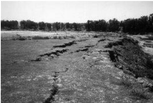
Figure 2.26 Lateral spreading (El Asnam, 1980).
