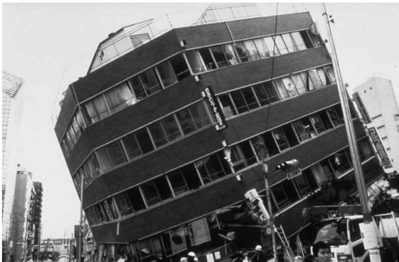
Figure 2.28 Bearing capacity failure due to liquefaction (Hyogo-ken Nambu earthquake, 1995).
