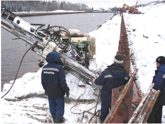
Fig. 1 Experimental works on Volga-Baltic Channel
