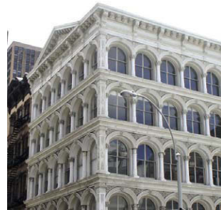
A 19 th century cast-iron facade in New York City.
