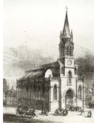
An early concrete building: Le Vesinet, 1864, by Francois Coignet.
