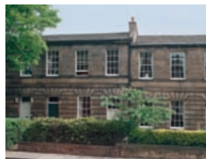
504 Stucco terrace of large Italianate houses, c. 1840. The stucco would originally have been stone-coloured but brightly coloured paints became from the 1960s onwards a sign of gentrification. Notting Hill Gate, West London.
