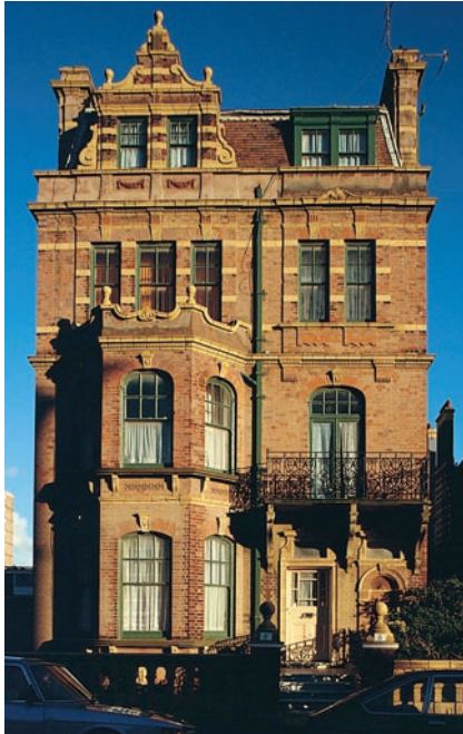
14 Brick house; Charfield, Gloucestershire; c. 1885.
