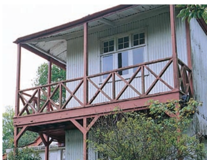
172 Iron porch with corrugated iron roof on terrace; Beccles, Suffolk; late 19C.
