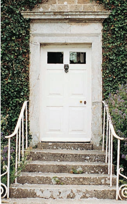
219 Six-panelled door with lights (probably inserted later); Chilcombe, Dorset; second half of 18C.
