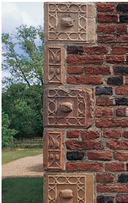
513 Terra-cotta cresting on gatehouse, ornamented with dolphins, egg-and-dart and guilloche patterns; Layer Marney, Essex; c. 1520.
