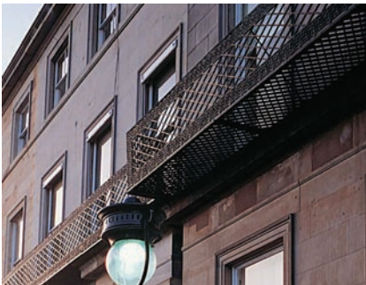
37 Iron balconies and canopies on terrace; Cheltenham, Gloucestershire; c. 1815–20.
