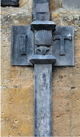
416 Lead downpipe and fixing, cast with heraldic scallop shell and initials; Stanway House, Chipping Campden, Gloucestershire; 16C.
