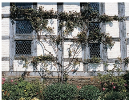
522 Cruck frame on medieval cottage; Osmaston, Derbyshire.
