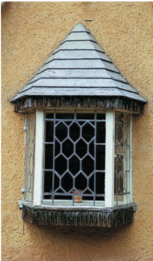
333 Wooden glazing bars on Gothick-style sash window; Stout's Hill, Uley, Gloucestershire; 1743.
