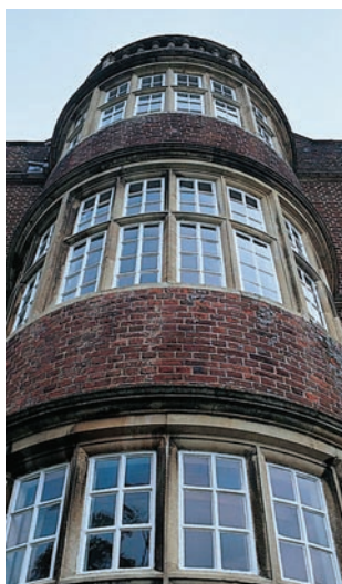
559 Bay with stone mullion casement windows on manor house: Lytes Cary, Somerset; 1533.
