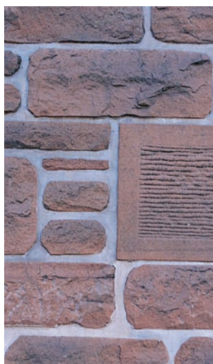
473 Sandstone with granite snecking; Port William, Dumfries and Galloway.
