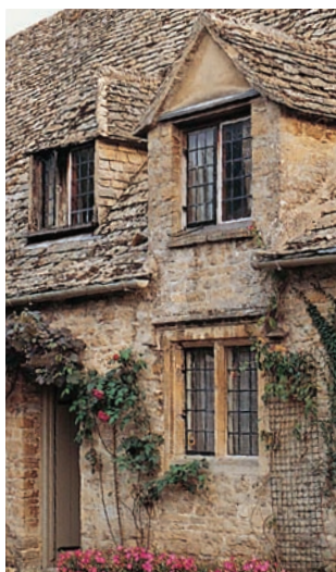
606 Oriel window on manor house; Great Chalfield, Wiltshire; late 15C.
