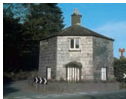
406 Tollhouse facing in three directions, each marked with a bargeboarded gable. Built c.1831 when Bruton Turnpike took over new road to Frome. Bruton, Somerset.
