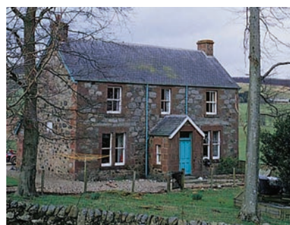
287 Small thatched stone farmhouse; this has a 1602 datestone on the chimney stack. Such stones often marked an improvement or addition and it is likely that some of the building is earlier. Stockland, Devon.
