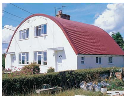
174 Corrugated iron porch roof and cottage roof; Mudford, Somerset.
