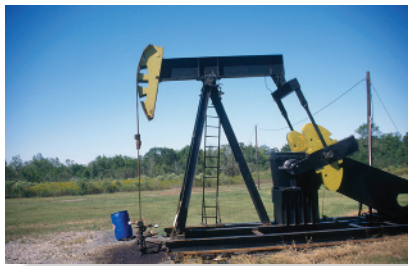
Engineers must account for possible fatigue failure of the moving parts of this oil-pumping rig.
