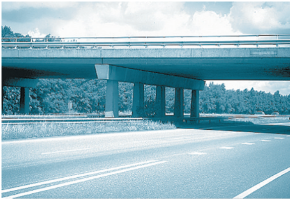
An example of a statically indeterminate beam used to support a bridge deck.
