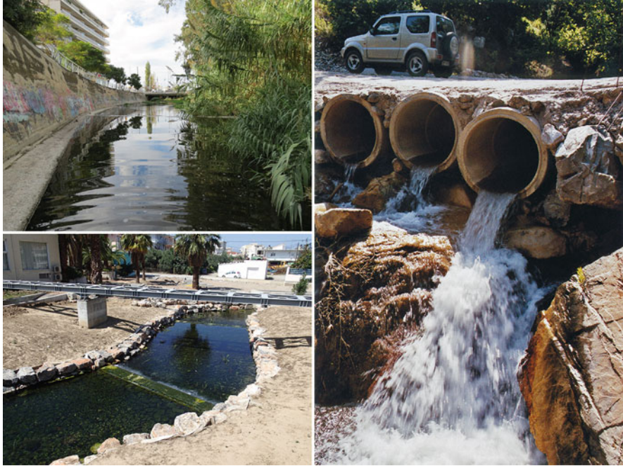
Fig. 3 Challenges for restoration ecology in Greece (clockwise from top left ): urban stream restoration, the flood-prone area of the Pikrodaphne stream in the Metropolitan Athens basin; road culvert creates artificial fish barrier in the Erymanthos river basin, Peloponnese; poorly designed urban spring-fed river park creation at the town of Skala, Peloponnese (Photos: S. Zogaris)
