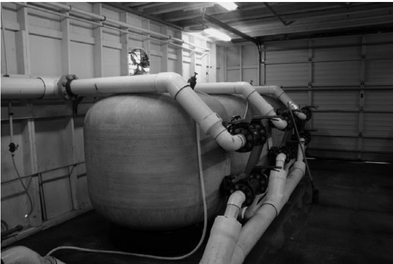
Fig. 2.21. Large sand filters can be used in both flow-through and recirculating systems to remove suspended solids from the water.
