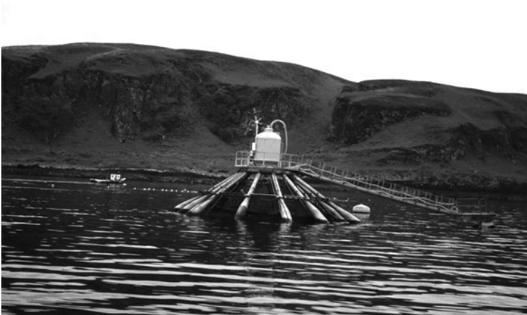
Fig. 2.28. A marine net pen in Scotland that was designed for offshore rearing of Atlantic salmon. While this net pen is located in a bay, it is exposed to the open ocean and has withstood waves as high as 5-6 m.
