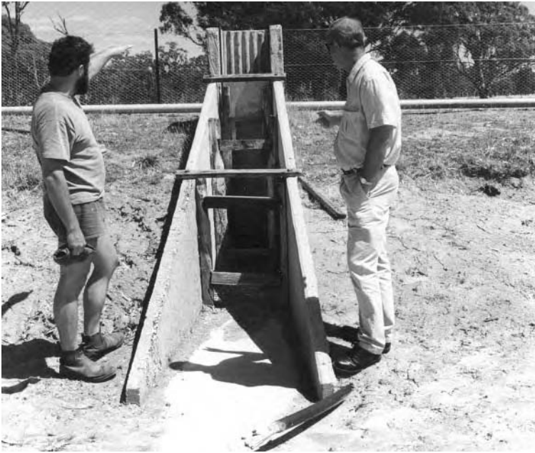
Figure 11.4. A simple in-bank monk that can be installed at the same time the pond is built.
