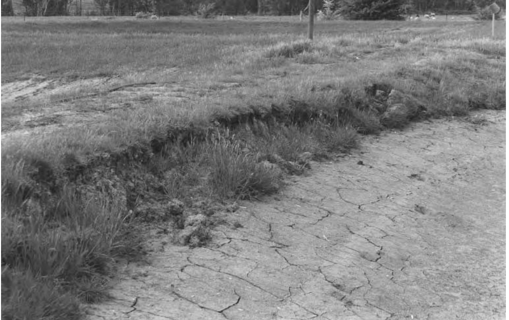
Figure 11.7. Wave action from aeration and wind will erode the banks until they form a natural batter of 1:3, so why not start at that point?
