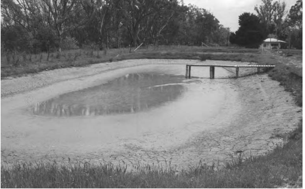
Figure 15.2. The advantages of having a well-designed and built pond are apparent on many scores, especially to break pathogen cycles. The results of not having bottom draining can be seen in this pond on an early yabby farm, built in the days when the industry emulated conditions found in productive farm dams.
