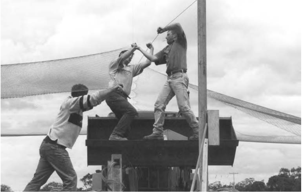
Figure 16.7. The penalty for not having the netting spread evenly along the wires is the impossible job of getting the threaded wires to meet at the cable.
