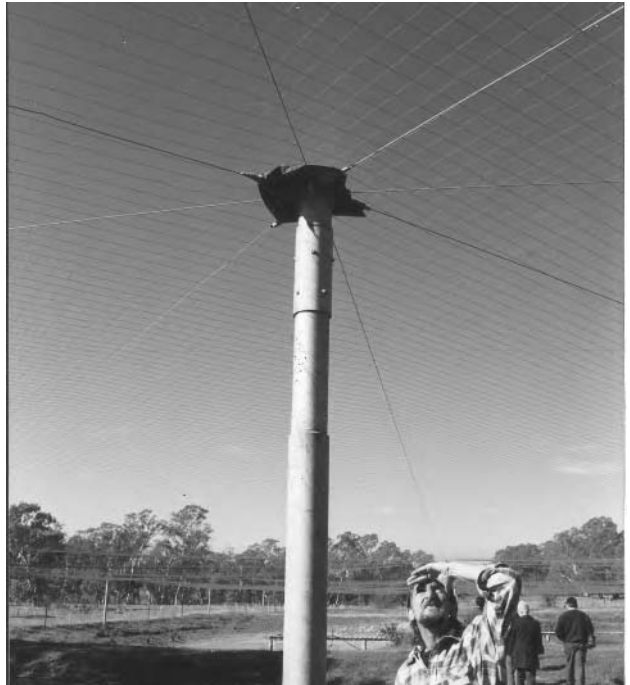
Figure 16.8. Well-erected netting will last for years and, if you have any sort of a crop to protect, will usually pay for itself in the first year. Note the steel posts and solid structure of this frame, a real engineer's job.
