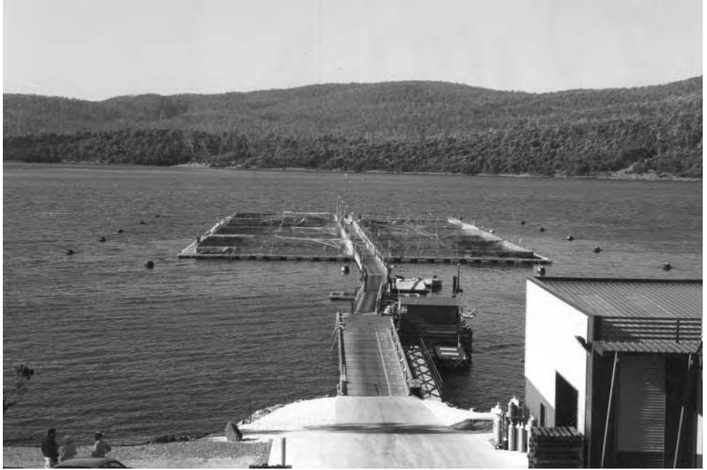
Figure 2.1. Floating cages come in all sizes and shapes, from these large salmon cages to small fresh-water-based production cages of <10\text{m}^3 . Shown here are the cages of a shore-connected salmonid farm on the Tamar River in Tasmania. Note the easy vehicular access and automated food delivery conduits to each pen.
