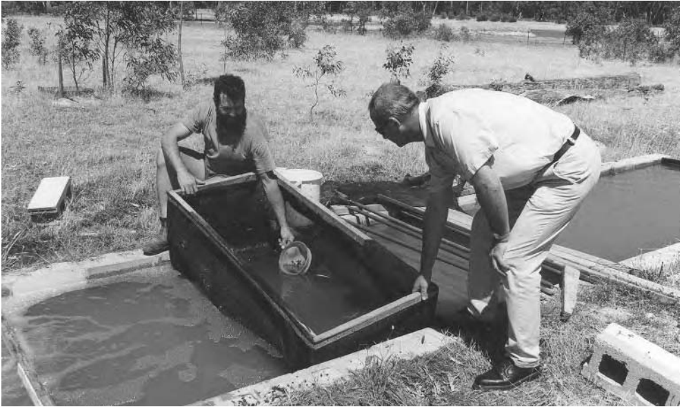
Figure 11.6. The external sump at Wartook Native Fish Culture. All the fry production ponds drain to this one ‘fish-out’ sump. Note the flat all-weather working area surrounding the sump.
