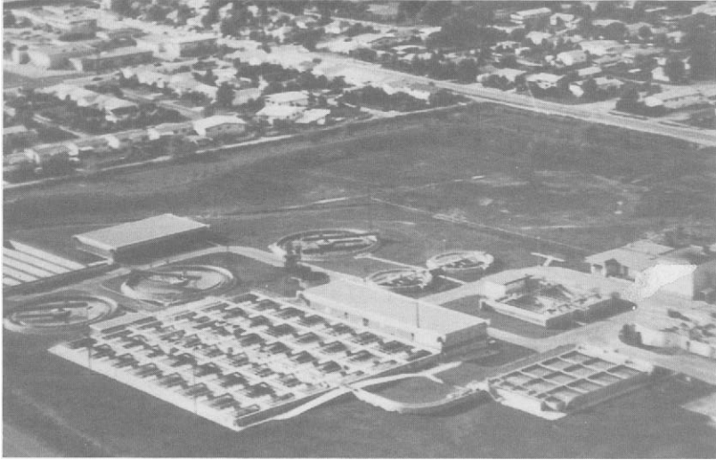
FIGURE 8–10. Aerial view of a secondary wastewater treatment plant. [Courtesy Envirex.]
