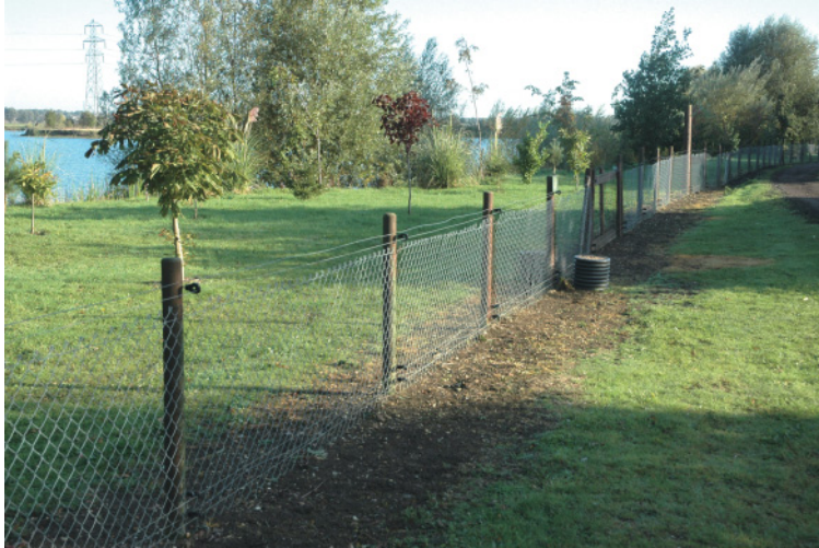
Figure 17.2 Electrified otter fence.
