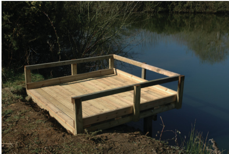
Figure 10.23 A finished cantilevered fishing platform.
