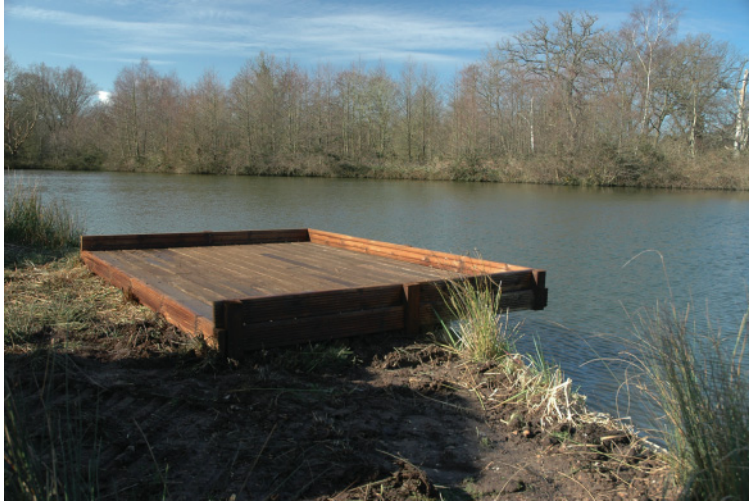
Figure 10.21 A cantilevered platform.
