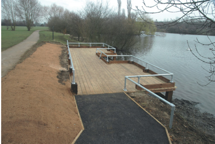
Figure 10.24 A platform with walkway.
