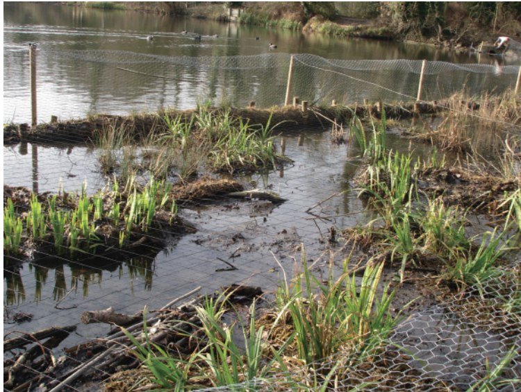
Figure 23.21 Pre-planted coir-fibre pallet installed in a pond margin.
