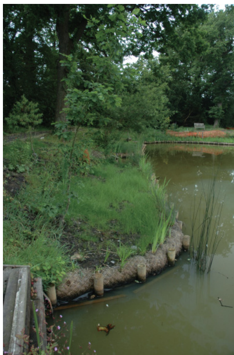
Figure 23.23 Pre-planted coir-fibre roll installed along a pond margin.
