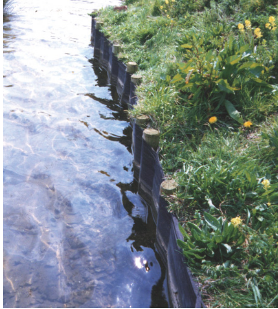
Figure 16.5 AGA Span nylon revetment curtain.
