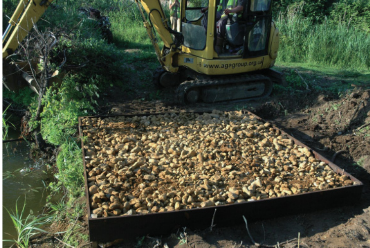
Figure 10.28 A finished granular fill swim.
