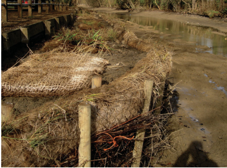
Figure 16.1 Backfill behind a coir fibre roll revetment.
