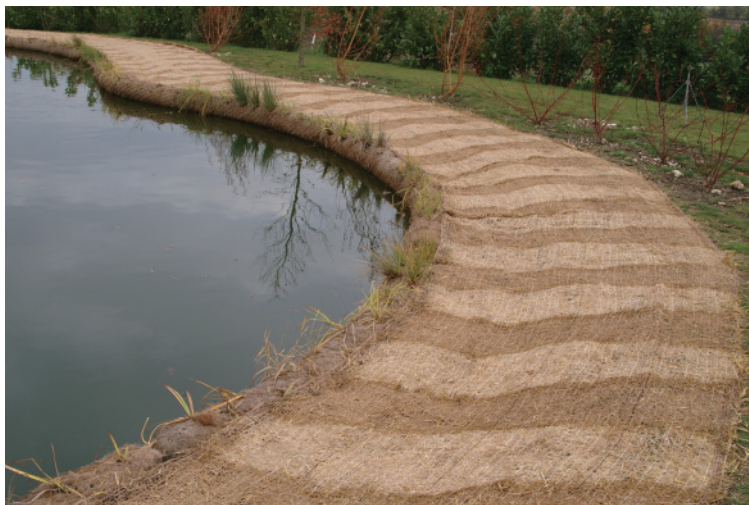
Figure 16.6 Turf reinforcement mats over a seeded bank.
