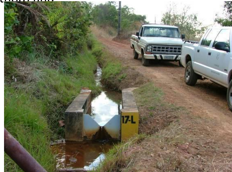
Fig Leakage measurement using a triangular weir gauge
