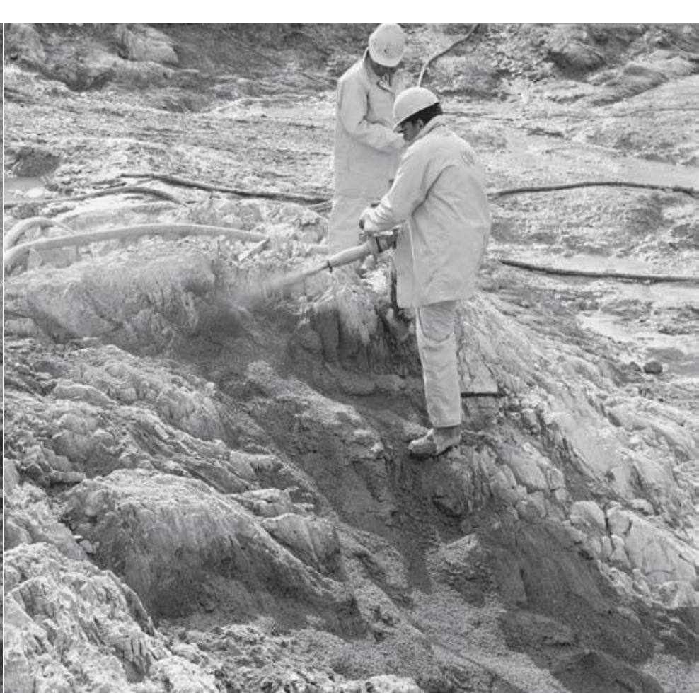
Application of pneumatically applied mortar on seams in the cutoff foundation
