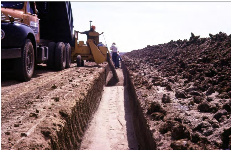
Trenching method – backfilling trench
