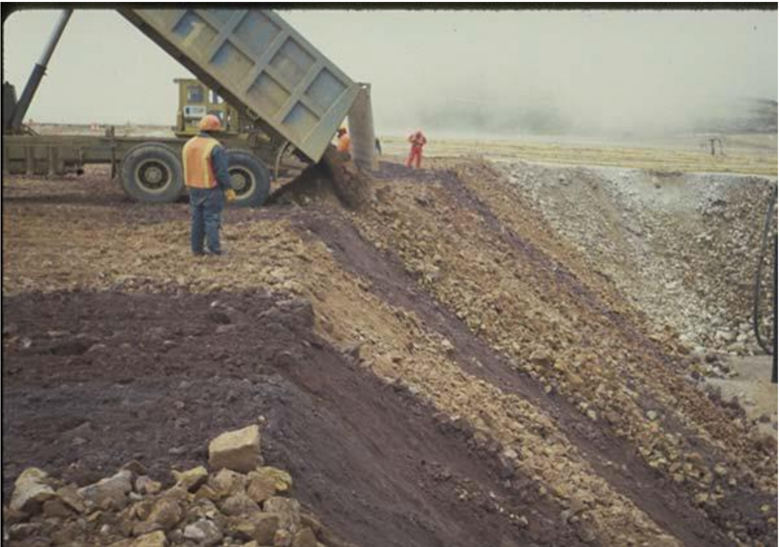
Rock dump loose lift placement in 45 ft (15 m) thickness
