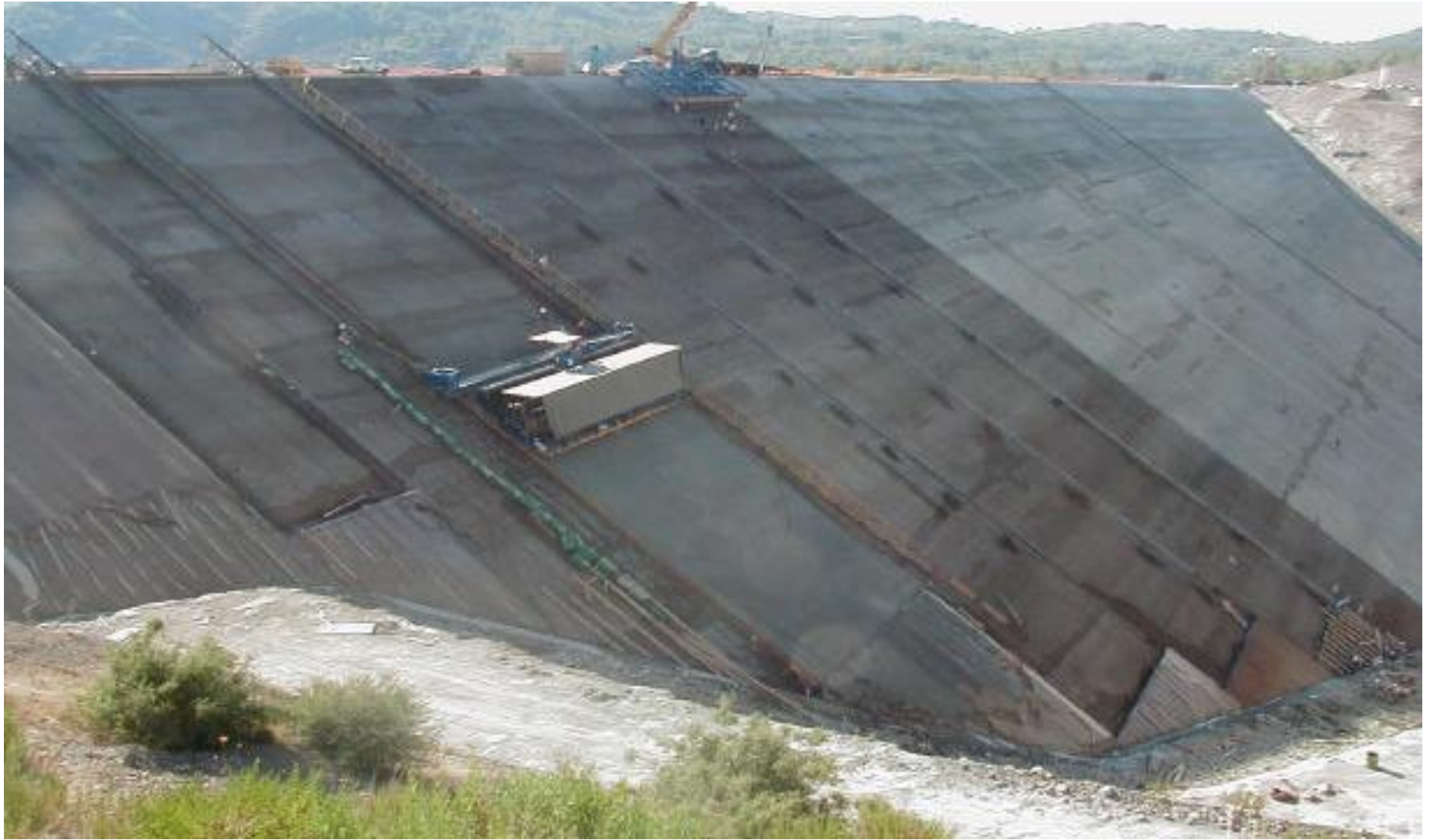
Upstream Face Slab Concreting
