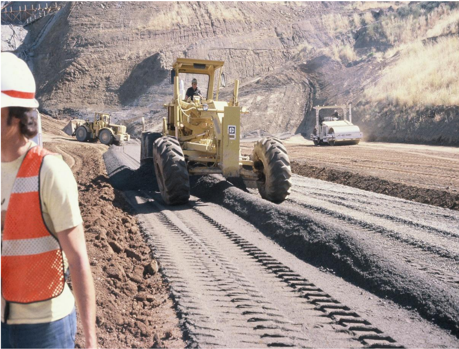
Spreading sand filter material ( usually accomplished by graders or dozers)
