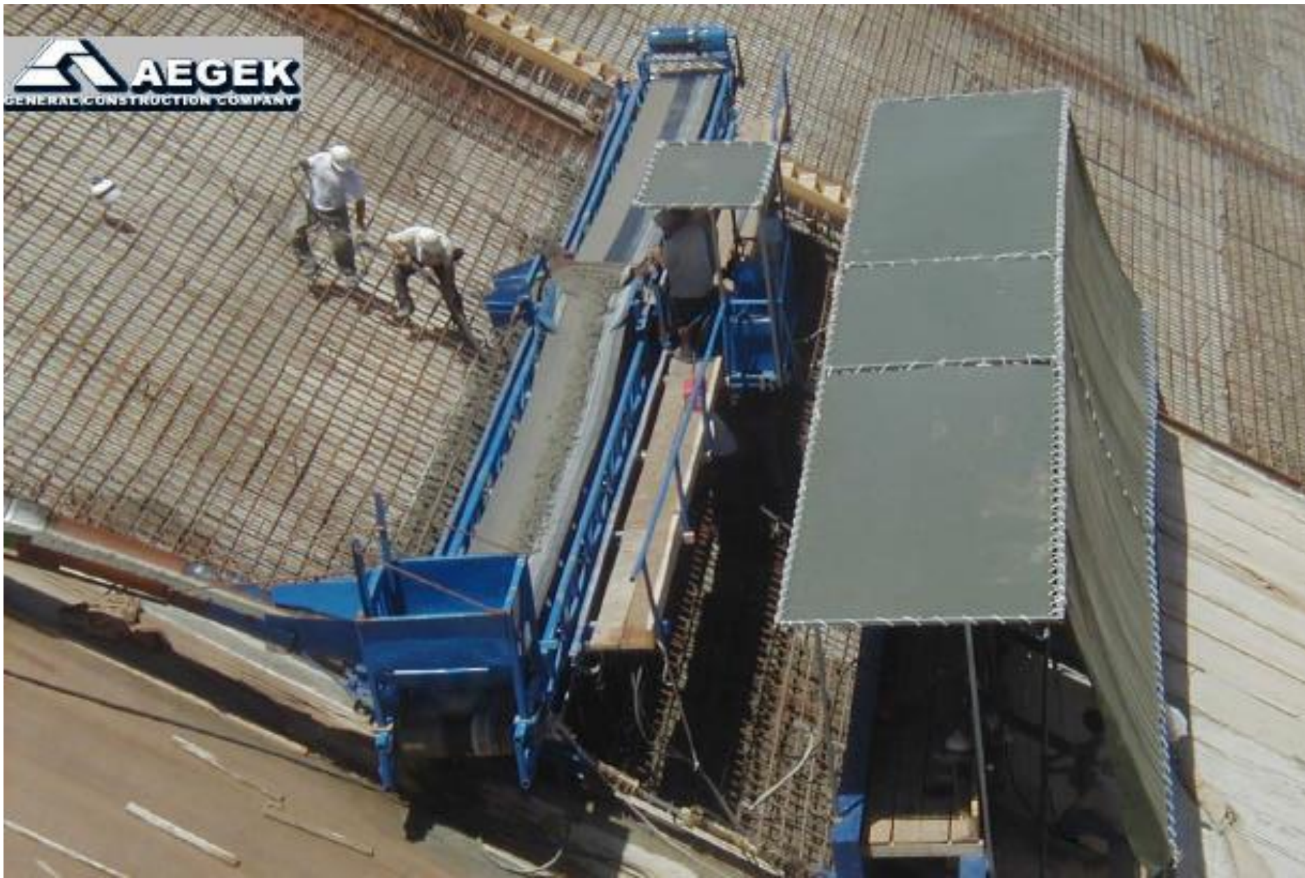
Self climbing slip form with side discharger
