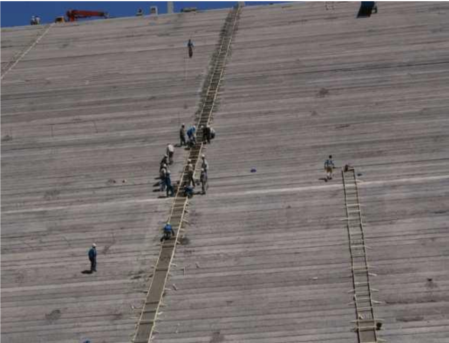
Placement of the mortar pads
