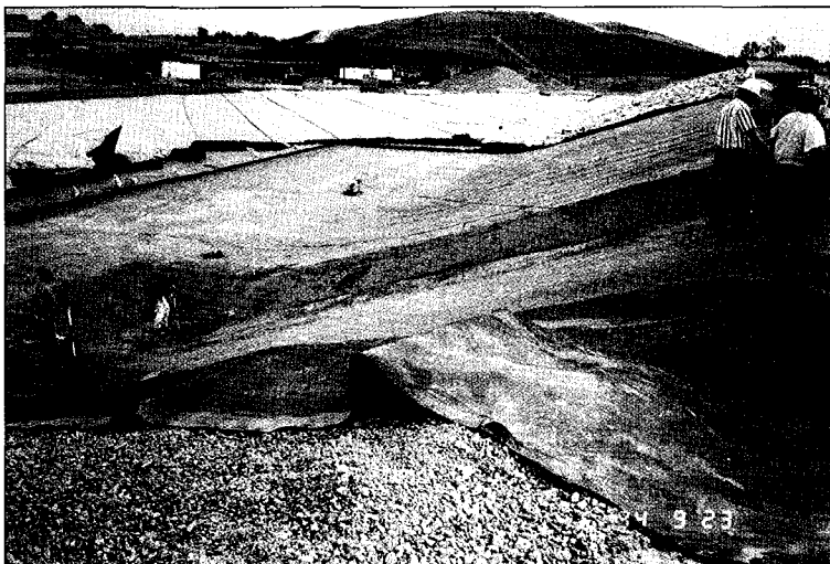
Part of the liner construction of a new landfill at the High Acres Landfill and Recycling Center in Fairport, New York. The hill in the background is a "closed" landfill, which has been through final cover.
