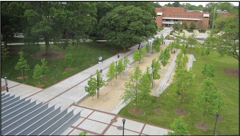
Photograph 31. Terraces that infiltrate stormwater with favorable safety characteristics (shallow steps and wide, good footing).
