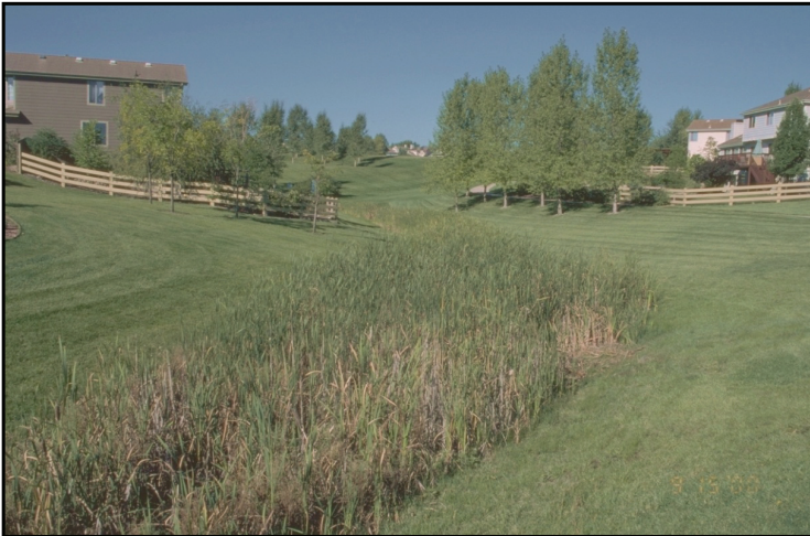
Photograph 23. Wetland swale integrates nicely into residential area and does not pose a significant safety risk to residents, since flows spread out and slow down and tall vegetation discourages access.
