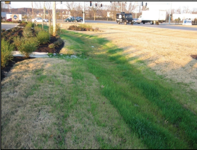
Photograph 28. Bioswales can provide significant hydrologic and water quality benefits while also being safe.
