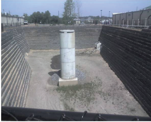
Figure 1. Dry Detention Basin with Safety Concerns Due to Steep Side Slopes and No Egress or Escape Route
