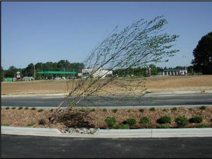
Photograph 34. Large trees in bioretention facilities should be staked for the first year for stability. These unstaked trees have become a hazard during a high-wind event.
