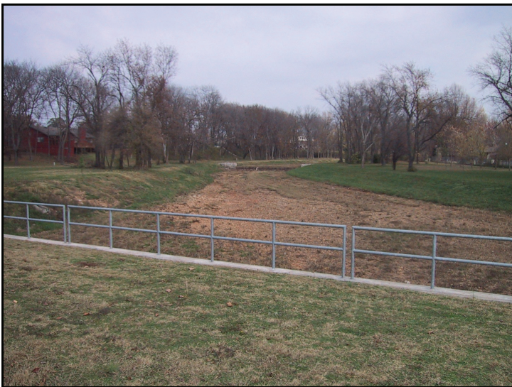
Photograph 42. Railings at elevated crossings of major drainageways are standard.
