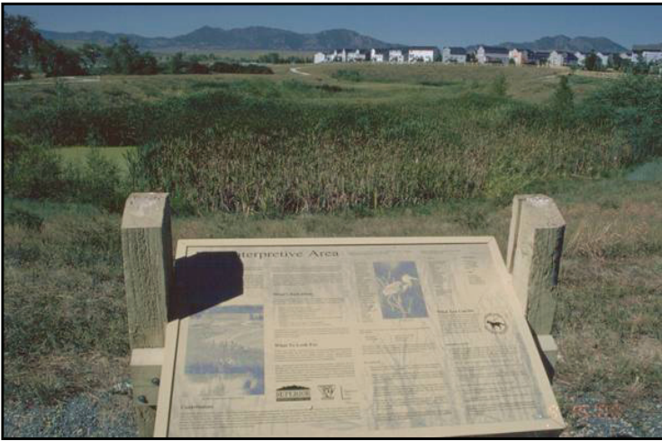
Photograph 22. Encouraging public education and access to stormwater facilities enhances public safety.
