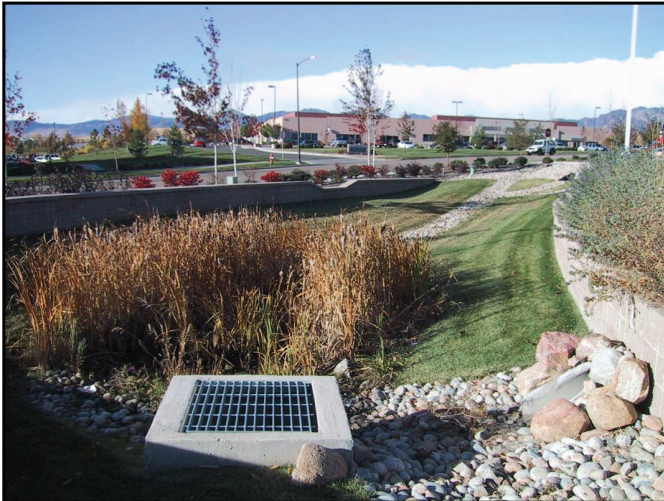
Photograph 14. Extended dry pond with mild side slopes, low retaining walls, shrubs discouraging access, good visibility and access, racks on outlet structures, wetland vegetation to discourage access to outlet and rock (cobble) on banks.
