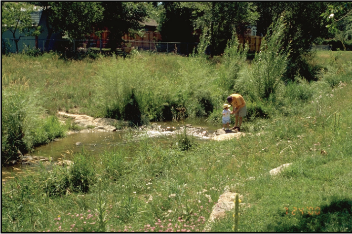
Photograph 37. Facilities like this bioengineered drainage channel with a low-grade control structure are attractive to the public and must provide good egress, mild slopes and solid footing.
