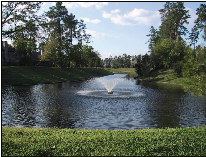
Photograph 18. Fountains help to maintain water quality and reduce mosquito problems by avoiding stagnant, quiescent water.
