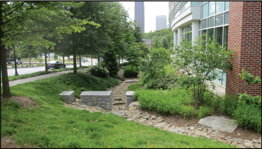
Photograph 41. Small channel with good footing, shallow design depth, low design velocities, grade control and good access.
