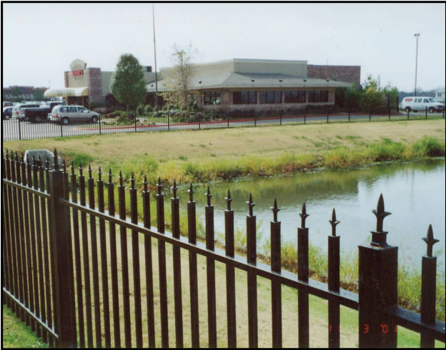
Photograph 19. Fencing is provided around retention pond, along with mild side slopes and good visibility.
