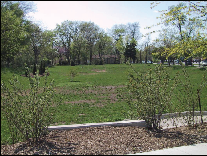
Photograph 17. Dry pond serves as park when it is not raining; it has mild side slopes and good visibility, is aesthetic and is well integrated into the neighborhood.
