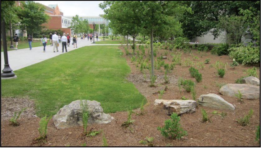
Photograph 30. An attractive bioretention basin with mild side slopes that has good access and visibility, and which drains well and interfaces nicely with the walkway.
