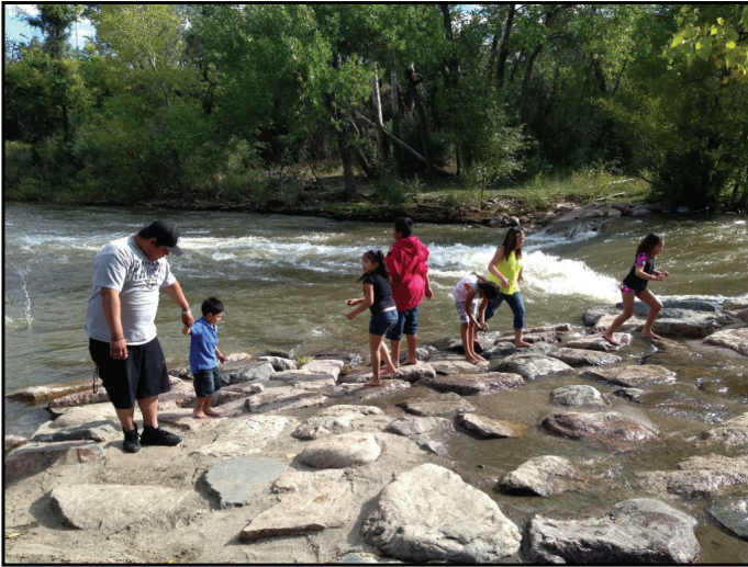
Photograph 51. Grouted boulder drop structure with safe hydraulic characteristics—essential given public use in area.
