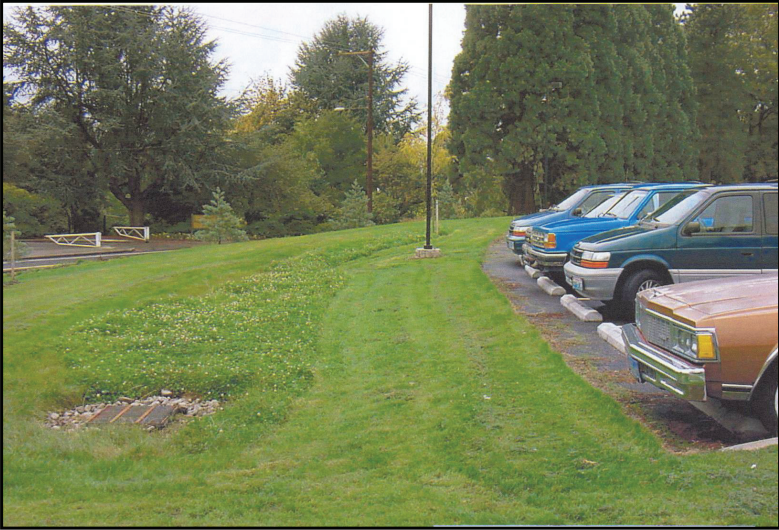
Photograph 39. Grass swale with mild invert slope and side slopes and shallow invert slope into grate.
