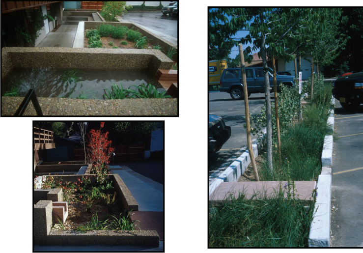
Photograph 26. These LID retrofits at an office building significantly increased onsite storage and infiltration compared to the traditional drainage facilities they replaced and are safe for building tenants and visitors.
