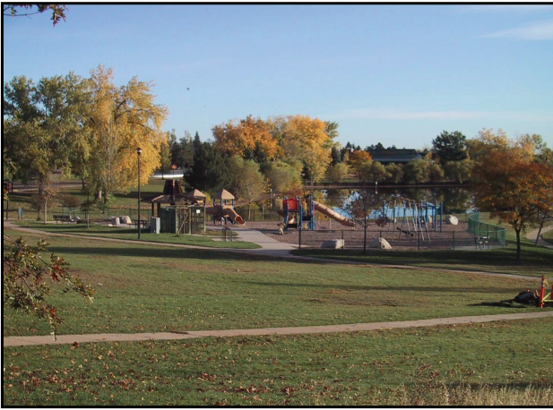
Photograph 13. In a retention pond next to a playground, the side slopes are very mild (approximately 10H:1V) both above and below normal water level.
