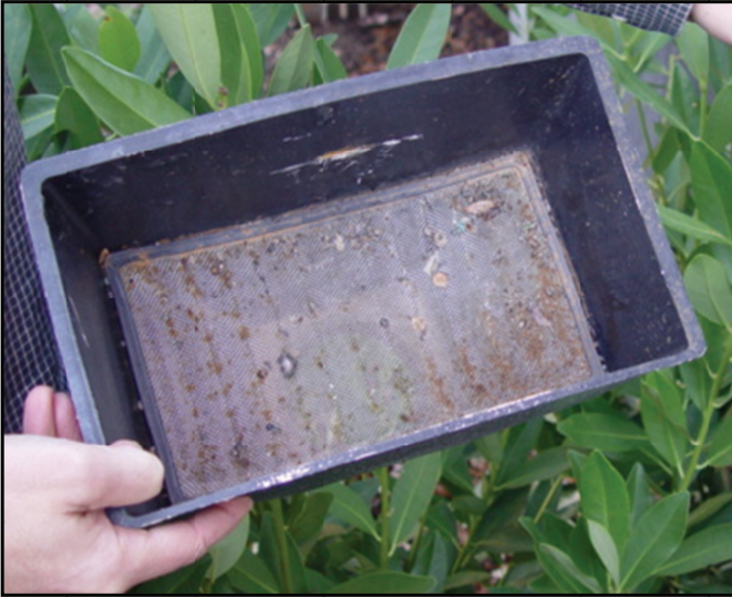
Photograph 36. Grit filter in a rain harvesting system with mesh that is too fine for adult mosquitoes to pass through.
