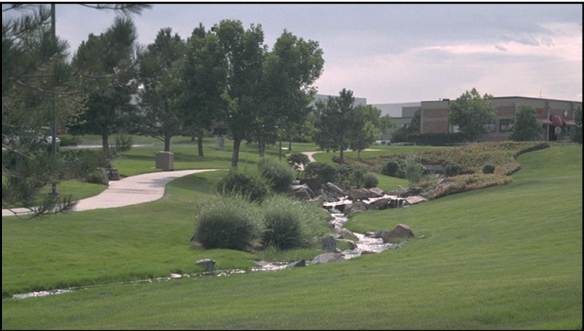
Photograph 38. At an engineered grass-lined major drainageway with a low-flow channel, a trail is set back far from the channel and higher than the 10-year flood elevation, and there is a mild side slope from the trail to the channel bottom.
