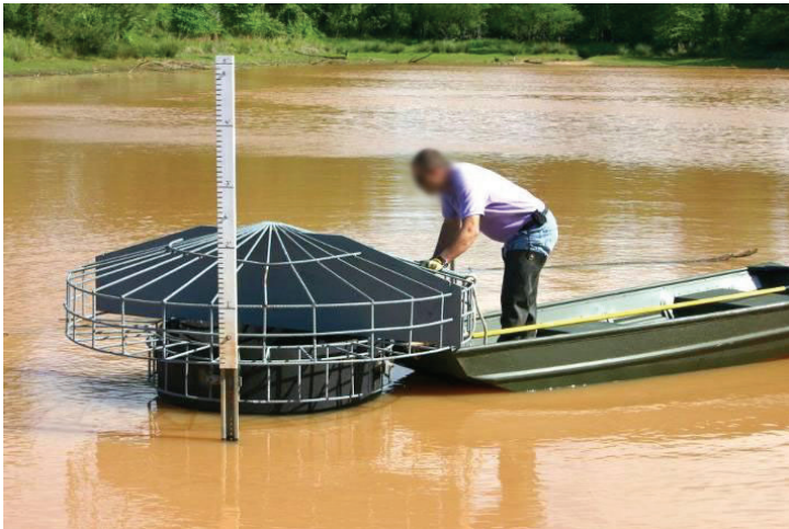
Photograph 6. A demonstration of four unsafe practices: This inspector (1) is alone in the boat, (2) is standing in the boat, (3) is not wearing a life vest, and (4) is wearing waders, which would act as an anchor if he fell in.
