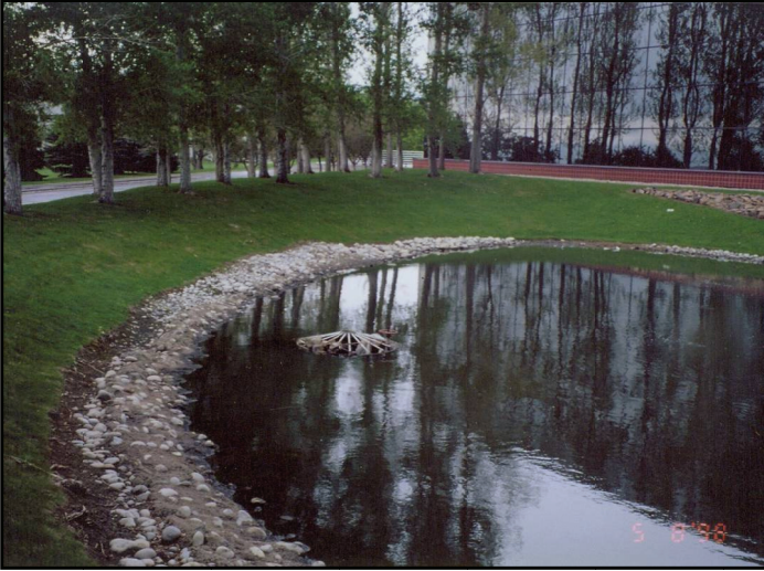
Photograph 15. Retention pond in office park with rack on outlet pipe, mild side slopes above and below the normal water surface, and good footing around edge.
