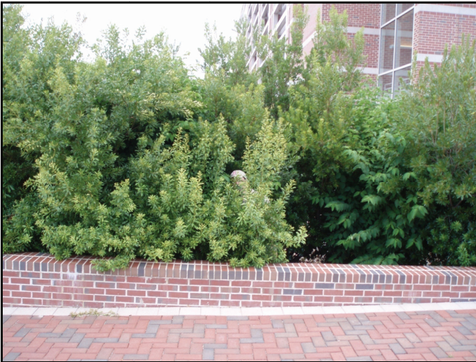
Photograph 33. Poor plant selection and lack of maintenance have resulted in an overgrown rain garden, which could provide cover for those with criminal intent, an obvious danger to passersby.
