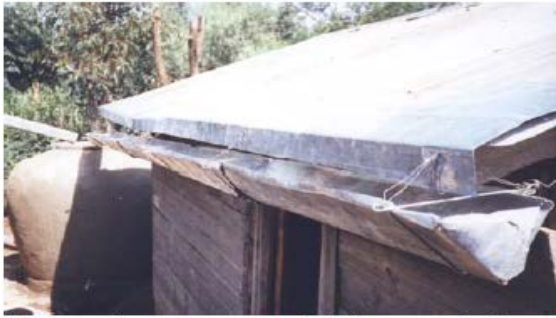
V-shaped gutter suspended from a splash-guard.
