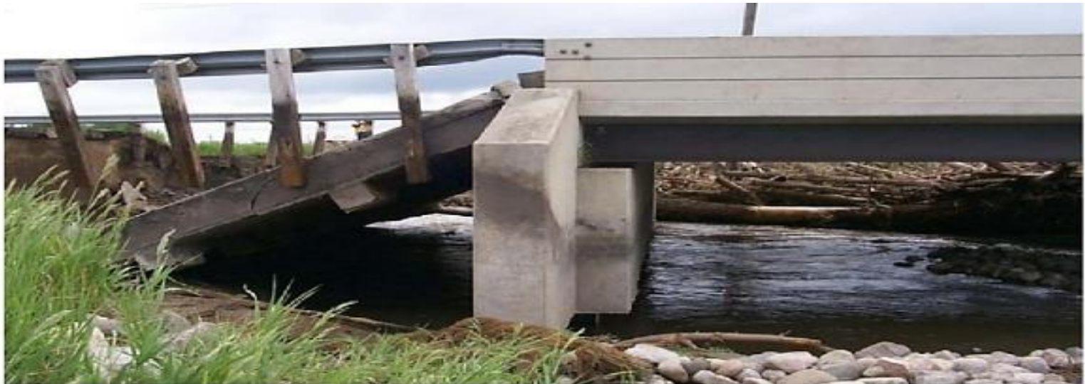
Fig. Abutment Fill Loss
