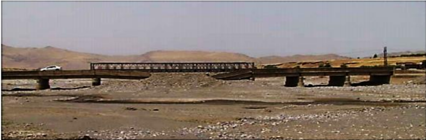
Fig. Zharawa Bridge was greatly damaged by flood. The bridge was subjected to foundation settlement, movement and displacement which resulted in cracks and concrete failure to several beams.
