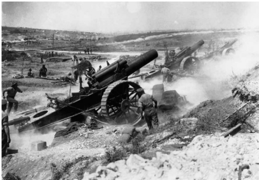
3 Artillery: the big killer. Battle of the Somme: British 8 inch howitzers of 39th Siege Battery, Royal Garrison Artillery in action in the Fricourt Mametz Valley, August 1916. Photo courtesy of the Imperial War Museum, London (Negative Number: Q 5818)
