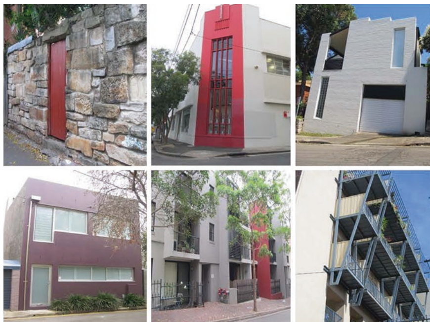
Plate 5.3 Chippendale—Main Planning Issue. Left to right Utilizing historic fencing; Converting factory to housing; Infilling new housing; Utilizing heritage colours in Infill housing; Medium density new housing; and, Converted building with new balconies added ( Source Raymond Rauscher 2009–2014)
