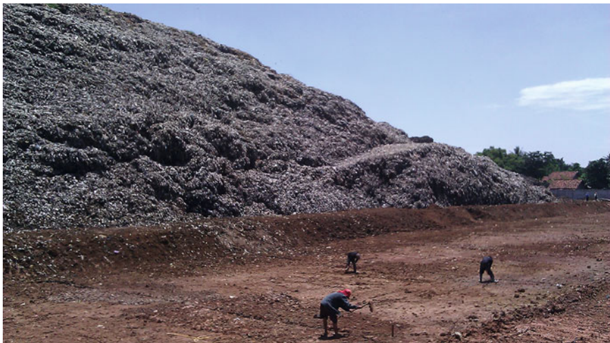
Fig. 12.3 Workers preparing the fifth zone of Sumur Batu landfill
