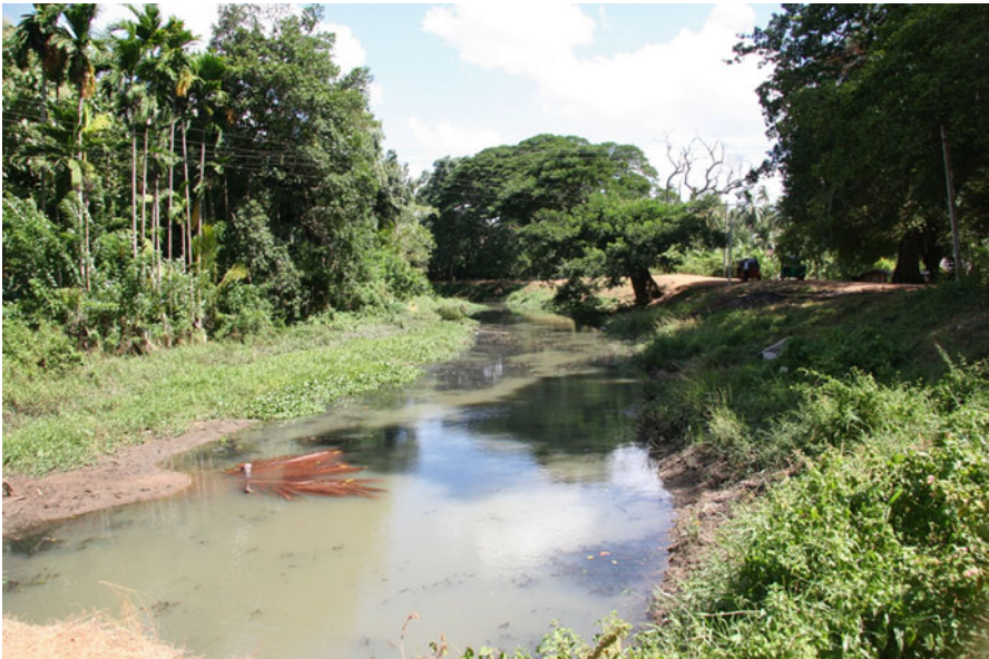
Fig. 8.10 An ancient feeder canal close to the modern one in Fig. 8.9, with a single bank that traps the local inflow and slow velocity as it is a contour canal that retains a large command area
