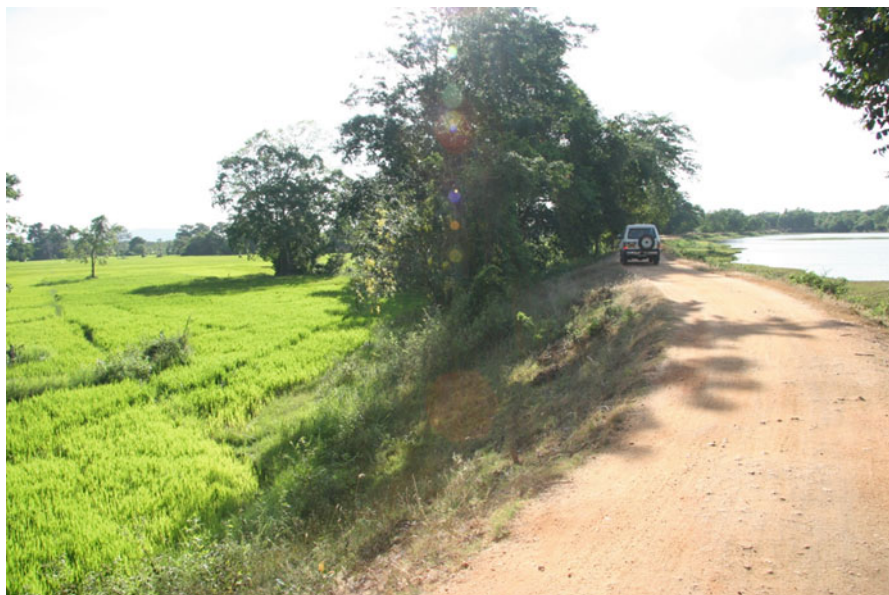
Fig. 8.6 Embankment of a tank
