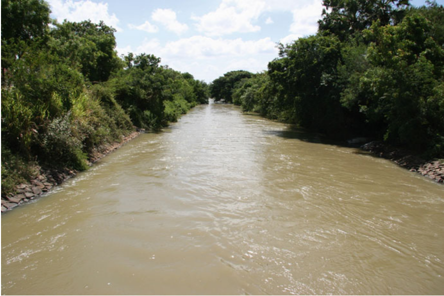
Fig. 8.9 A modern feeder canal with paved embankments on both side and steep gradient
