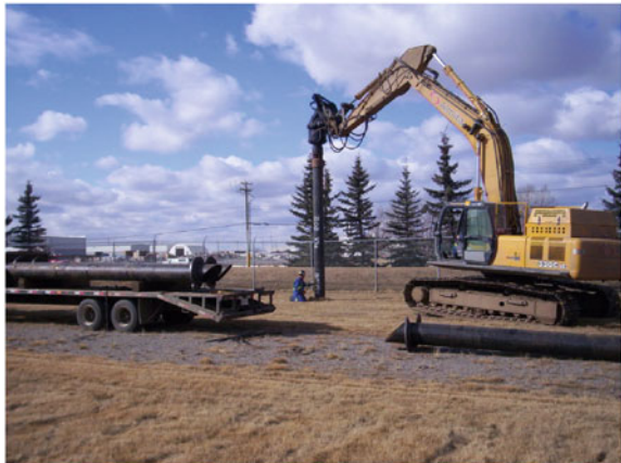
Fig. 12.9 One of a number of small wind turbine pile foundations being driven into the ground. The bevel on top of the foundation seen in the foreground is cut off before attaching the turbine baseplate. Photograph by Rob Falconer, Enmax Corporation
