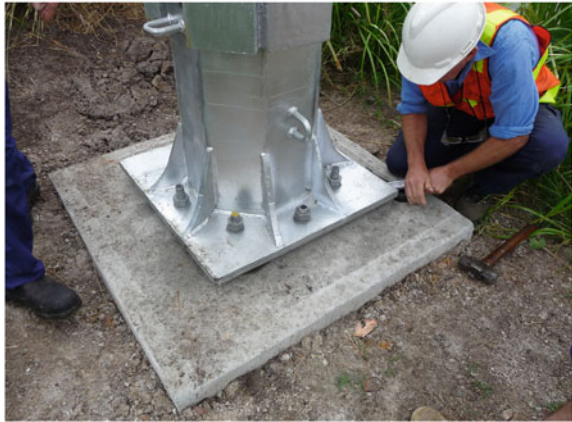
Fig. 12.8 Leveling a 5 kW wind turbine tower. This tower is hinged near its mid-height and can be easily swung up and down because the weights visible at the top of the photograph counter the weight of the turbine. Photograph by Paul Peterson
