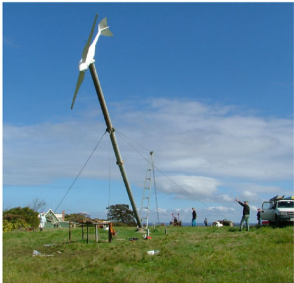
Fig. 10.10 A 5 kW turbine being raised on a guyed tower on French Island, Victoria, Australia
