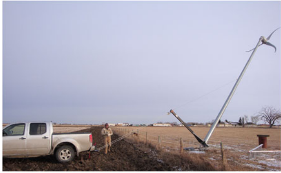
Fig. 12.7 A Skystream 2.4 kW wind turbine on a monopole tower being raised using a gin pole and winch attached to a four-wheel drive vehicle. Photograph by Rob Falconer, Enmax Corporation
