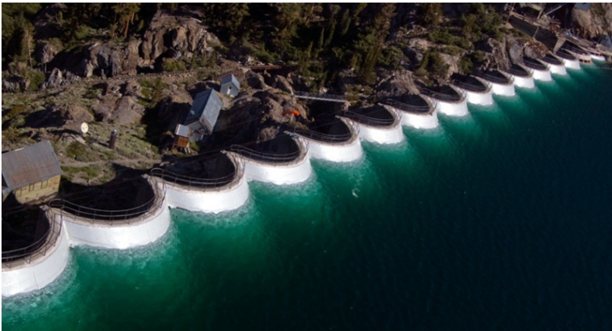
Figure 3. Upstream face (with geomembrane liner) of Gem Lake Dam.
