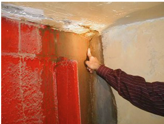
Fig. 2.11 Crack in concrete at draft tube door
