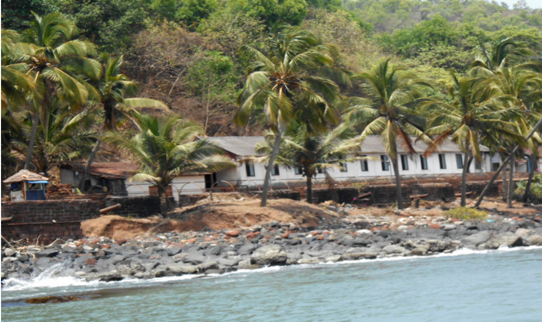
Fig. 10.13 Hard concrete structures adjacent to the HTL on the Goa coast ( 15^{\circ}29'5.0''\text{N} and 73^{\circ}47'40.4''\text{E} ) (Photograph taken on 04.04.2013 by Dr. Subhadra Devi Gadi (zoologist))
