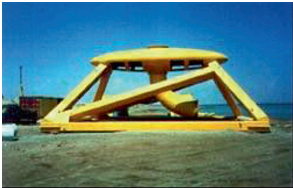
Figure 2. A submerged type of intake used to supply seawater feed to a desalination plant in Cyprus (Photograph courtesy of IDE Technologies)
