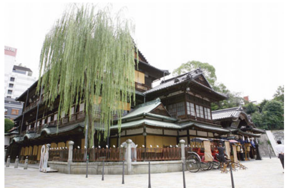
Fig. 12 The model indoor hot springs resort Dogo Onsen (Arima type hot spring), Ehime Prefecture
