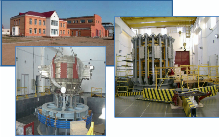
Figure 3. General view of KTM complex and installation of KTM on a workplace
