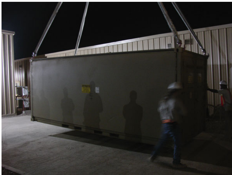
Fig. 2.5 Isoshelter containing a CT being carefully lowered to a concrete slab by a crane during the move to the new hardened facility. These isoshelters can provide operating room environments, large equipment such as CT or plain radiography rooms, and clean laboratories. Photo by Dr. Les Folio
