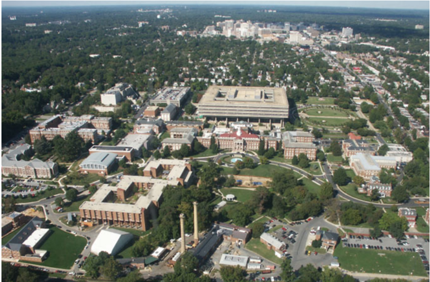
Fig. 2.2 Walter Reed Army Medical Center, a major Level 5 facility in the US. Photo by Dr. Les Folio
