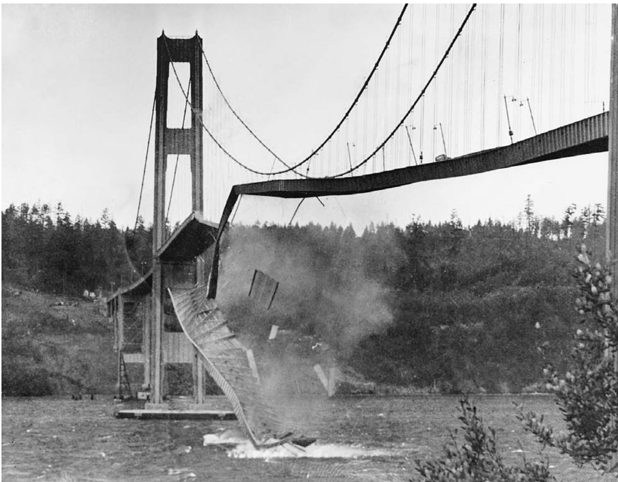
A large section of the concrete roadway in the center span of the Tacoma Narrows bridge crashes into the Puget Sound in Tacoma, WA, on November 7, 1940. High winds caused the bridge to sway, undulate, and finally collapse under the strain. Engineers use calculus derivatives to estimate the forces bridges must withstand. AP/WIDE WORLD PHOTOS. REPRODUCED BY PERMISSION.
