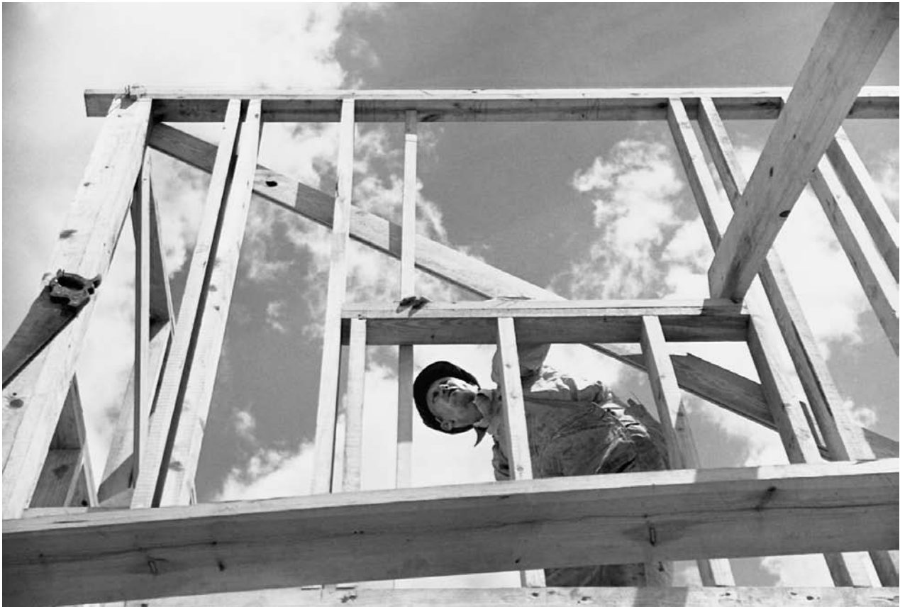
Carpenters use a variety of everyday math skills. CORBIS.
