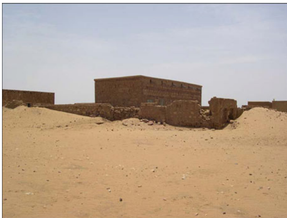
Photo. 13.1 Wind erosion around Banat village (photo courtesy S. Walker, August, 2005)
