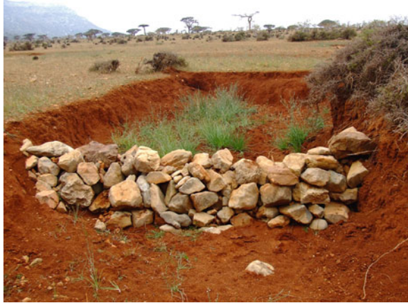
Fig. 29.6 Intact wall (W2)
