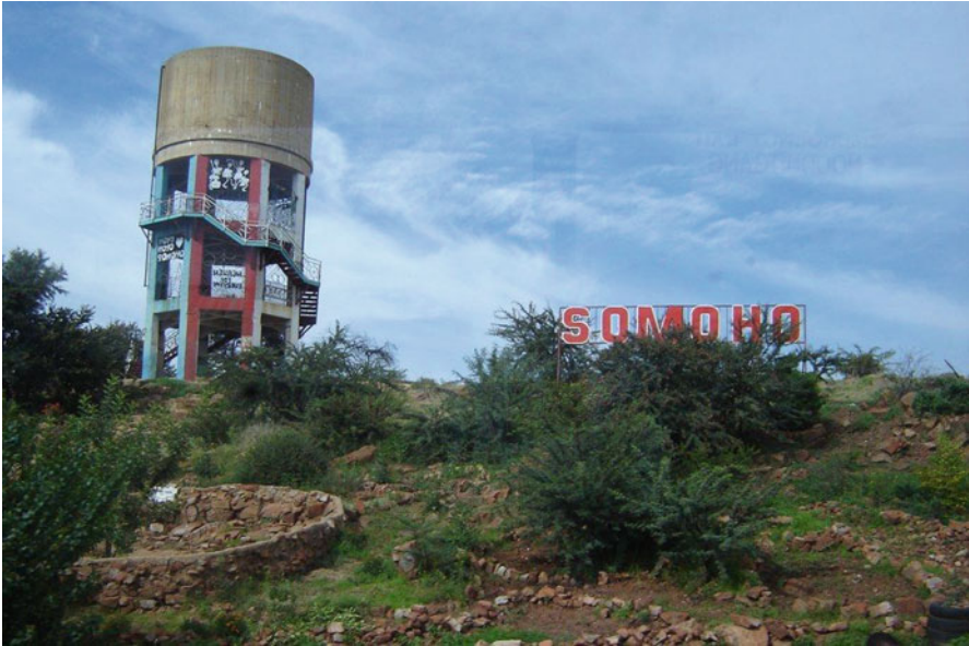
Fig. 6.1 Disused water tower decorated with art and dialogue circle in the forefront
