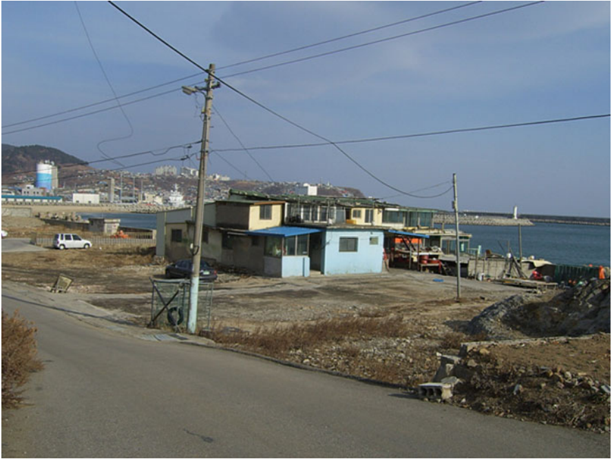
Fig. 12.2 Last remaining buildings in Bugok village. The houses had to be evacuated following Typhoon Rusa in 2002 (Photo by the Korean NGO Forest for Life )
