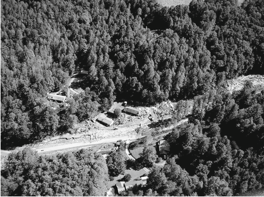
Fig. 9.1 Damaged and destroyed homes, and debris flow erosion and deposition along the run out zone (lower track) of the September 16, 2004 Peeks Creek debris flow in Macon County, North Carolina. The debris flow triggered by rainfall from Hurricane Ivan claimed five lives and destroyed 16 homes (September 19, 2004 NCGS photo). Refer to Fig. 9.17 for location
