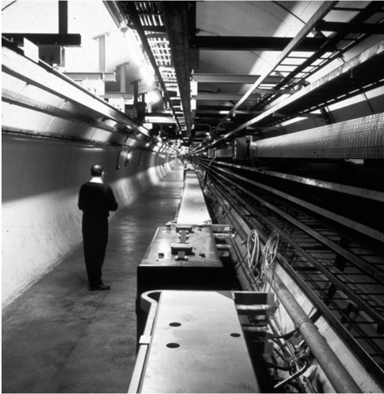
Figure 11.3. A view of the LEP tunnel. The beam travels in a pipe inside the multiple magnets that run down the centre of the picture. To the left is the track for a monorail that runs the length of the tunnel. To the right are various servicing and cooling ducts. (Courtesy CERN.)
