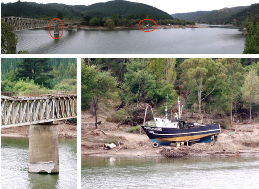
Fig. 1.1 Traces left by the 2010 Chile tsunami in the Maule River, Chile: a panorama of the river bend at about 7 rkm from the mouth, with views of a scoured bridge (zoomed-in, bottom left) and offshore fishing boats deposited by the tsunami onto a bared riverbank (zoomed-in, bottom right). Post-tsunami survey photographs, courtesy of Hermann M. Fritz, Georgia Tech
