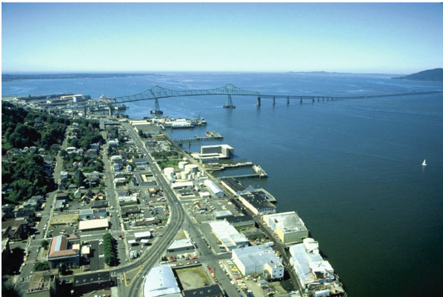
Fig. 1.3 View from Astoria, past the 6545 m long Astoria-Megler Bridge, toward the Columbia River mouth. Photo by Bob Heims, U.S. Army Corps of Engineers [Public domain], via Wikimedia Commons. August 1986
