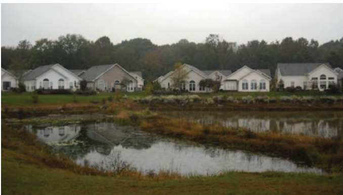
Fig 1 A constructed wetland in a residential development in Centreville, Maryland, USA. This wetland has been designed to permanently retain water. It is an example of one of the most accepted and effective best management practices for treating stormwater runoff and removing harmful nutrients. (© Paul Leishnam)
