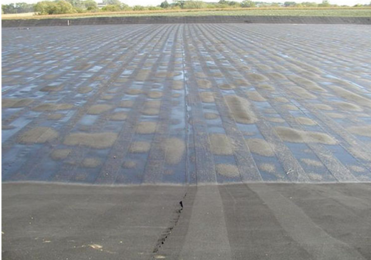
Fig. 5.4 Floating permeable cover installed on an earthen lagoon containing swine manure (Photo: Baumgartner Environics, Inc.)
