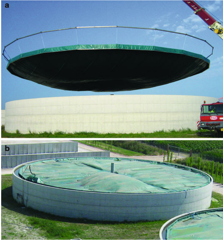
Fig. 5.3 A floating cover developed within the EU Agro Biogas project designed by Ecomembrane S.R.L. The photos show it (a) being installed, and (b) in use on biogas effluent tanks (Photo: B. Amon)
