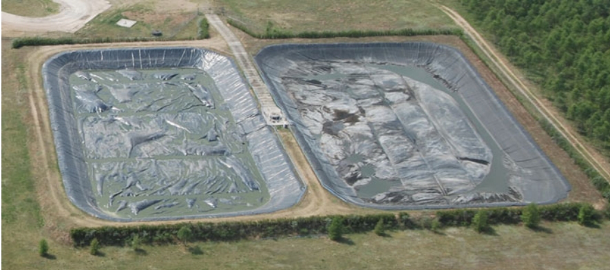
Fig. 5.2 Plastic covers on earthen basins in Poland (Photo: From archives Poldanor S.A.)
