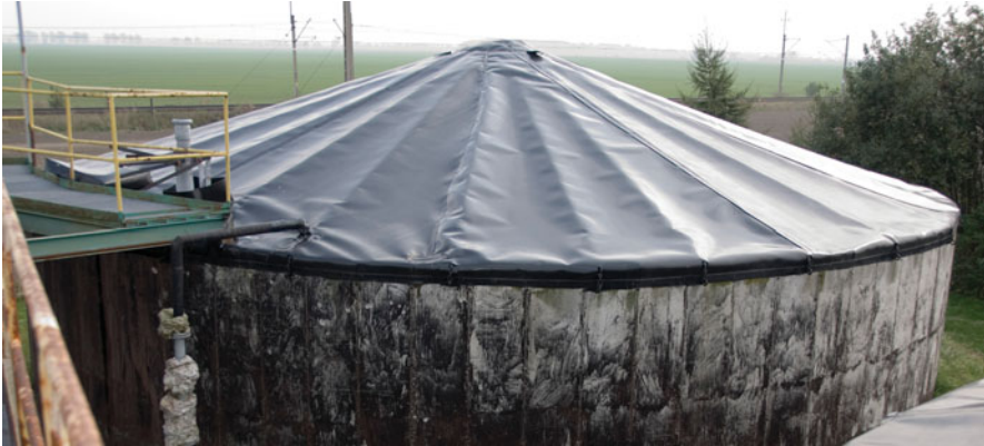
Fig. 5.1 Retrofitted tent cover in Poland (Photo: T. Kuczynski)
