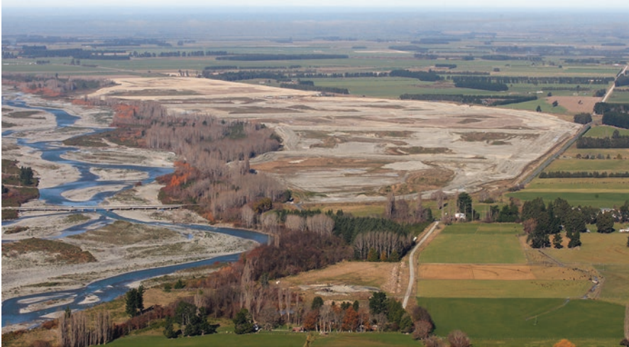
Fig. 3.13 Off River Storage adjacent the Rangitata River under Construction (John Bisset)
