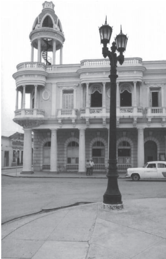
FIGURE 4.3. Palacio Ferrer sits at the western edge of Parque Martí in the heritage site of Cienfuegos. Built in the early 1900s by a wealthy sugar baron, José Ferrer Sirés, it is unique because of the blue mosaic cupola and spiral staircase. Famous opera stars, such as Enrico Caruso, who sang at the nearby Terry Theater, purportedly stayed at the Palacio Ferrer during visits to Cienfuegos.
