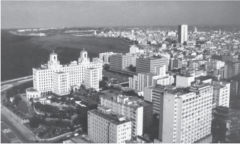
FIGURE 5.4. Hotel Nacional (center left with two towers), located on the Malecón, was built in 1930 and anchored the rise of Vedado in Havana’s “new” section, in contrast to Havana’s old quarters (top center).
