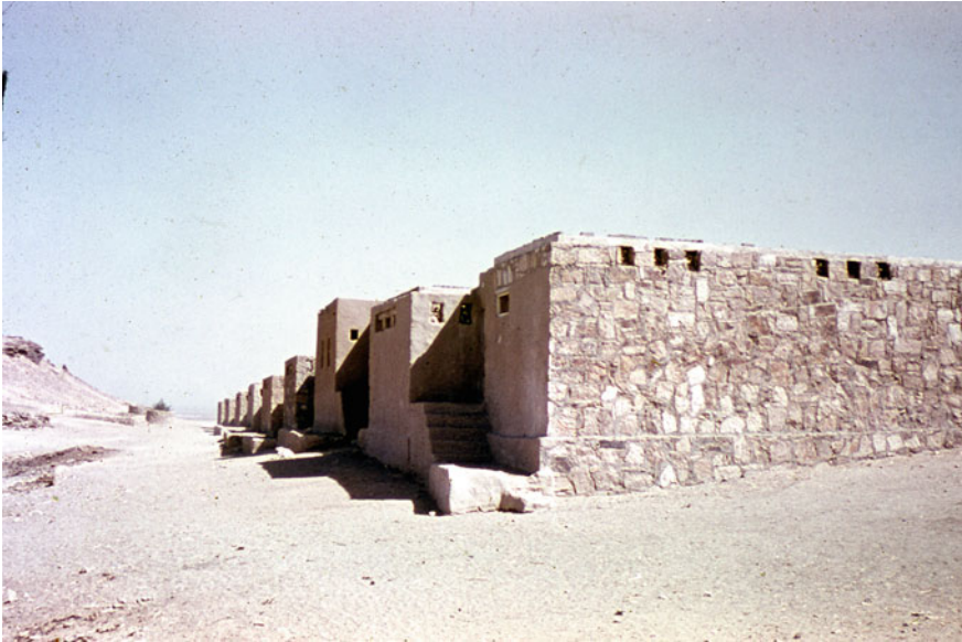
Fig. 7 Line of attached Nubian resettler houses with concrete roofs in Kom Ombo
