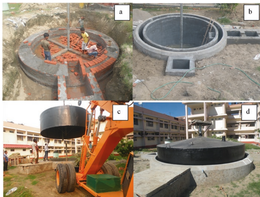
Fig. 1 (a–d) Construction phase of the biogas plant
