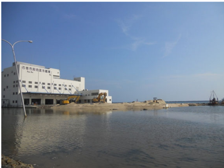
Fig. 5.12 Raising the level of Ishinomaki Port (Miyagi Prefecture in Japan) following the subsidence caused by the Great Eastern Japan Earthquake and Tsunami of 2011 . This clearly showcases how the raising of a coastal area that has been “submerged” by a natural hazard (in this case land subsidence due to an earthquake) does not result in the land being considered as artificial. To the authors’ knowledge, nobody has questioned whether this area is still part of Japan, or whether the baselines should retreat as a result of this subsidence
