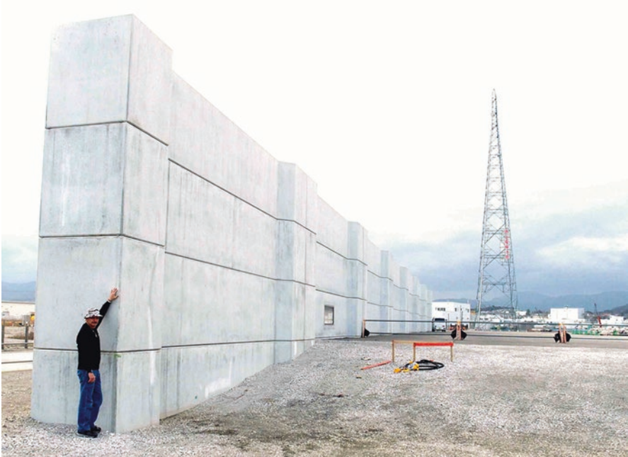
Fig. 18.2 Vertical seawall constructed nearby Kesennuma Fish Market (Miyagi prefecture) (Photo taken by the V. Santiago-Fandino in May 2016)
