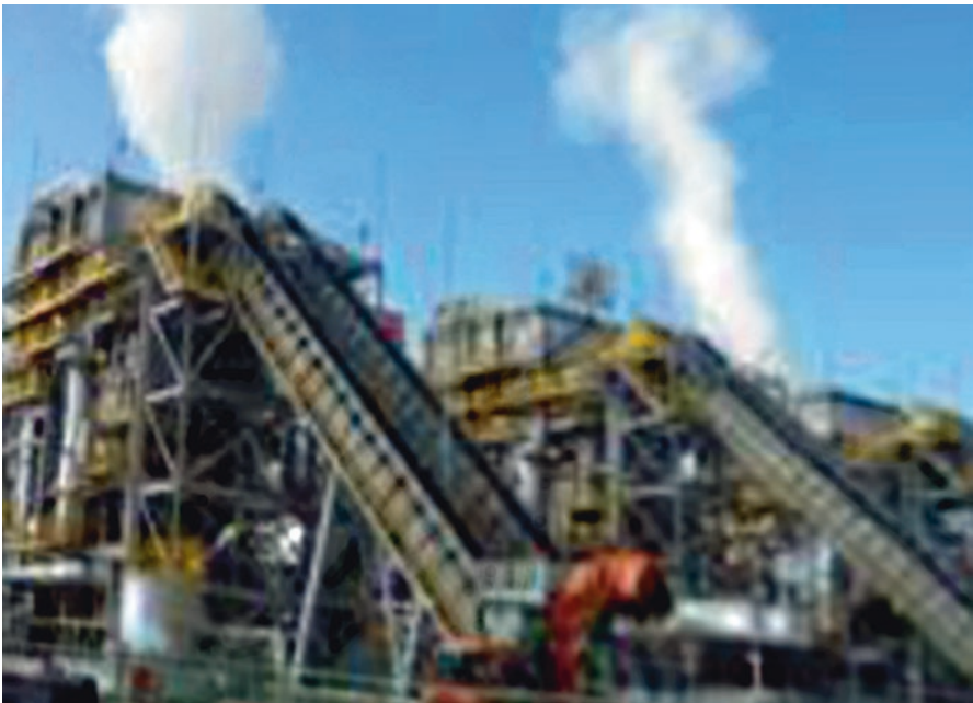
Fig. 5.7 Debris Operation site in Ishinomaki, Miyagi (IRP 2013)
