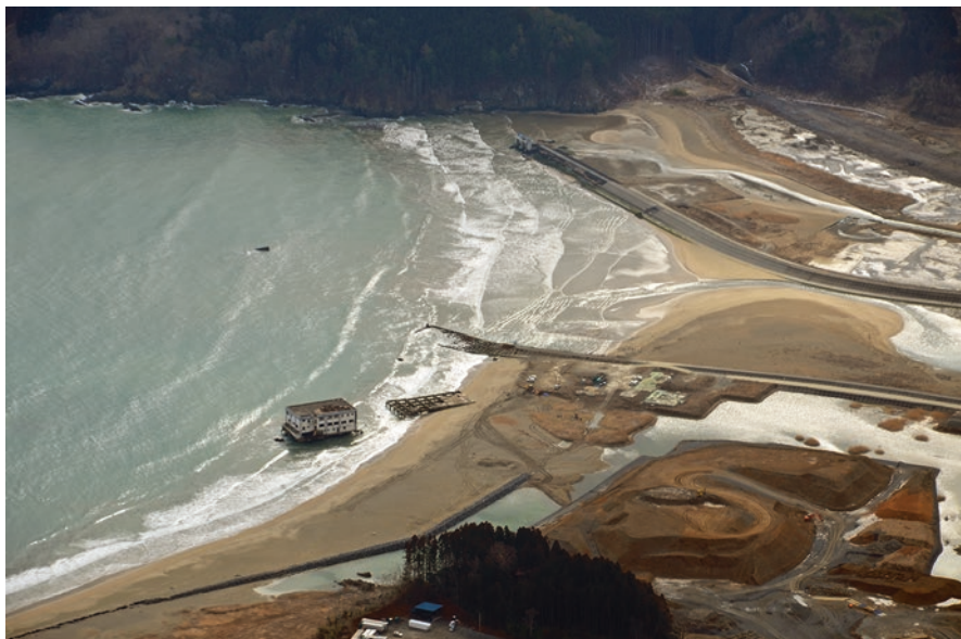
Fig. 18.3 Aerial view of a section of Kesennuma coast showing reconstruction works as well as evidence of the large coseismic subsidence (Photo taken in February 2015 by E. Mas during a joint reconnaissance flight with the Sendai Coastal Division of the Ministry of Land Infrastructure and Tourism (MLIT))
