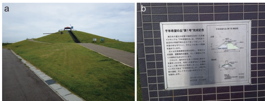
Fig. 14.2 Millennium Hope Hills, Iwanuma, Miyagi Prefecture (see Fig. 14.1a for location). (a) Artificial hill built with recycled concrete debris and rubble from the earthquake and tsunami. The hill can also serve as evacuation area (the top is 11 m above mean sea level). The black arrow on the left points to the sign indicating the height of the 2011 tsunami (Photo Kazuhisa Goto); (b) Plaque at the bottom of the hill showing the design of the hills and indicating that they were constructed using tsunami disaster waste, including concrete debris and tsunami deposits (Photo Catherine Chagué-Goff)
