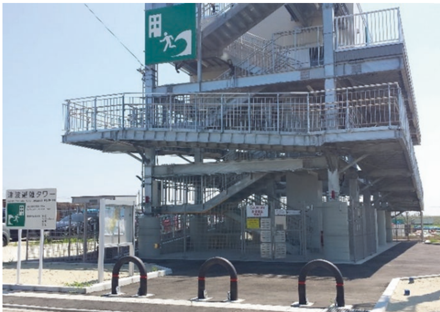
Fig. 5.16 Ido Tsunami Evacuation Tower (Photo by T. Norton Aug. 2016)
