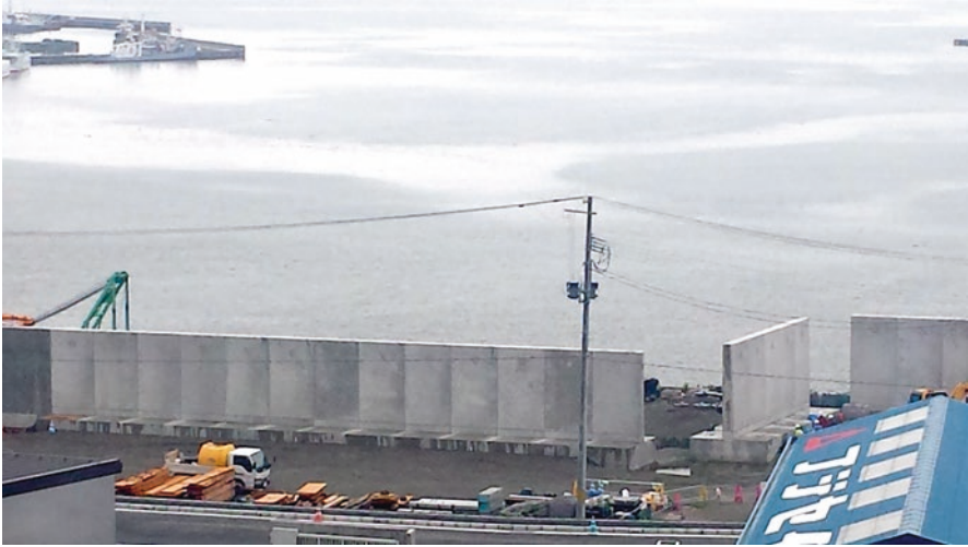
Fig. 5.23 Seawall being constructed in Kamaishi City (Photo by T. Norton Aug. 2016)
