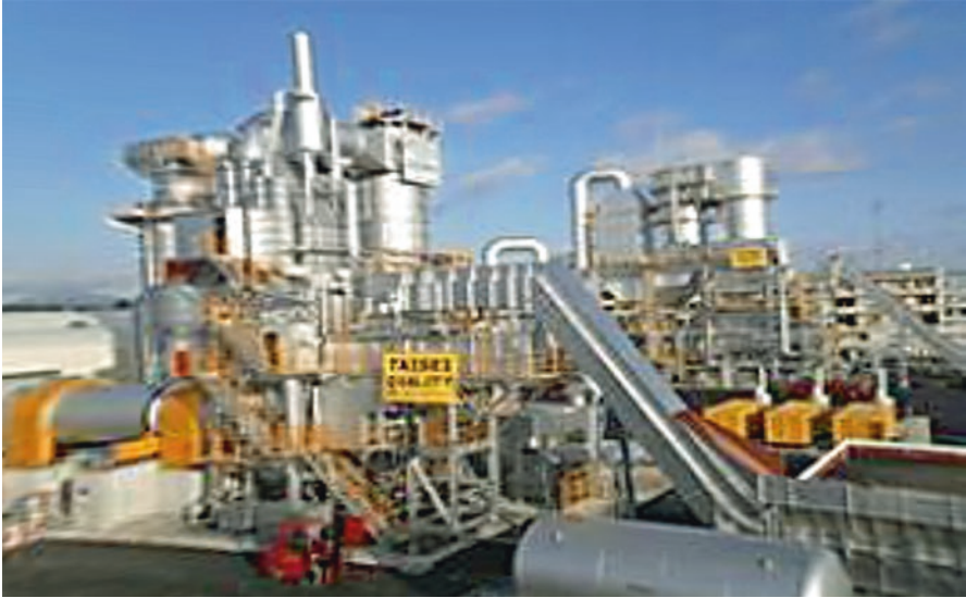
Fig. 5.6 Temporary incinerator in Kesennuma City, Miyagi (MOE 2012)
