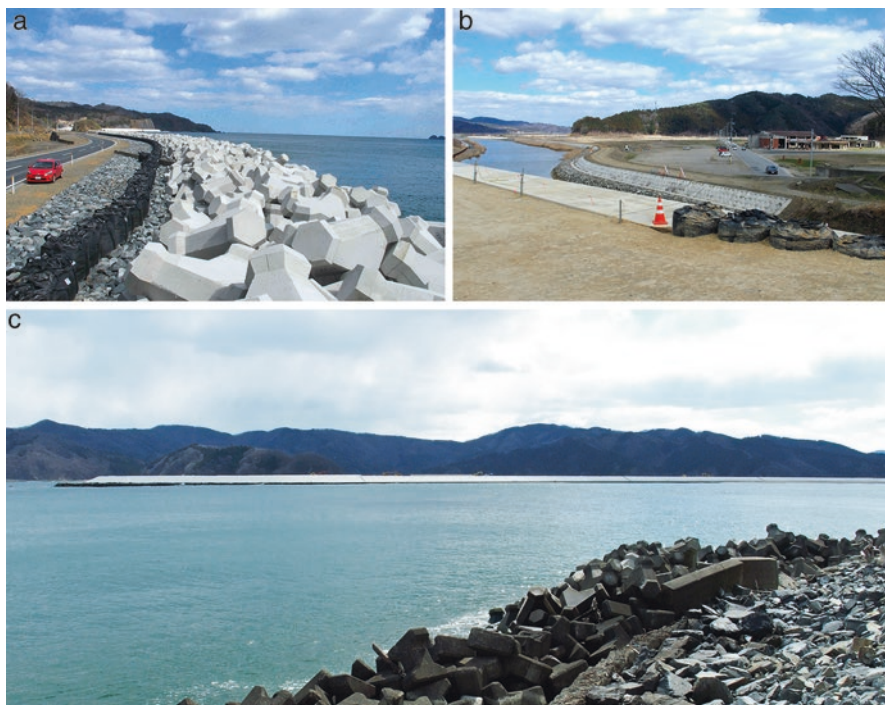
Fig. 18.6 Old Kitakami river (a) estuary seaward view; (b) works by the former Okawa school; (c) upstream view from the estuary and wall (Photos taken in March 2016 by V. Santiago-Fandino)
