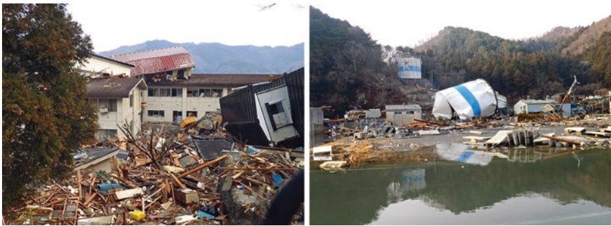
Fig. 17.3 Left: debris accumulated on 12th March at the back yard of the Field Center. Right: heavy oil tank displaced from the hill flowed out to sea (March 13, 2011) (Pictures taken by Yoshiyuki Suzuki; Tohoku University)
