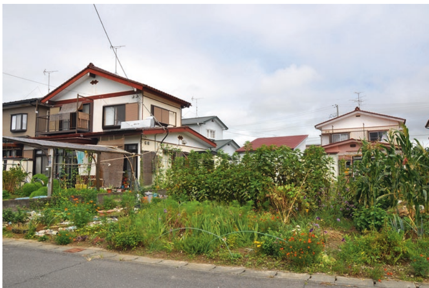
Fig. 10.7 Transformation of built environment in Ookaido-district, Ishinomaki. Photo and field survey data by author in August 2016
