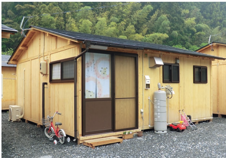
Fig. 11.1 Wooden temporary housing in Sumita Town
