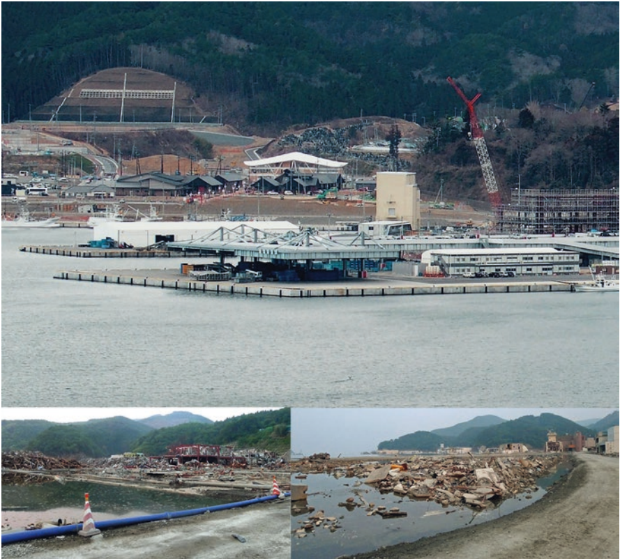
Onagawa Port in Miyagi Prefecture. This composite picture shows below the enormous destruction suffered by the port due to the 15 m high tsunami waves which destroyed more than 70% of the buildings and produced a large number of casualties. The top image gives a view of the extent of its reconstruction by August 2015 initiated by the local private sector and the community soon after the tsunami occurred; the ongoing large landscaping and over 4 m high ground rising to relocate commercial and industrial facilities can be easily seen (photos by V. Santiago-Fandiño)
