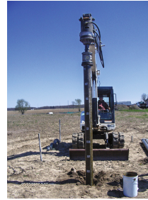
Fig. 6. FRP-G-HSP installation
