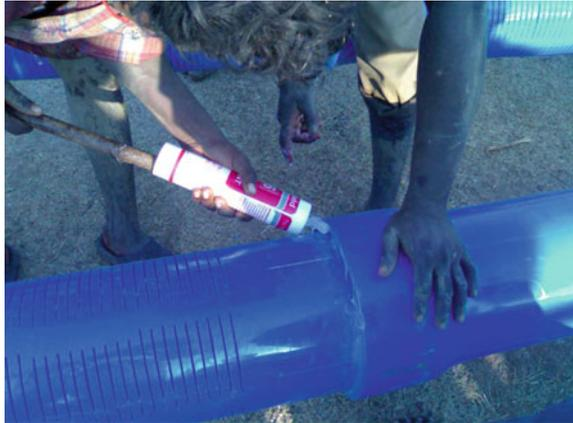
**Fig. 4.24** Untreated damaged casing in the well leaves a conduit to contaminate the fresh water bearing aquifer
