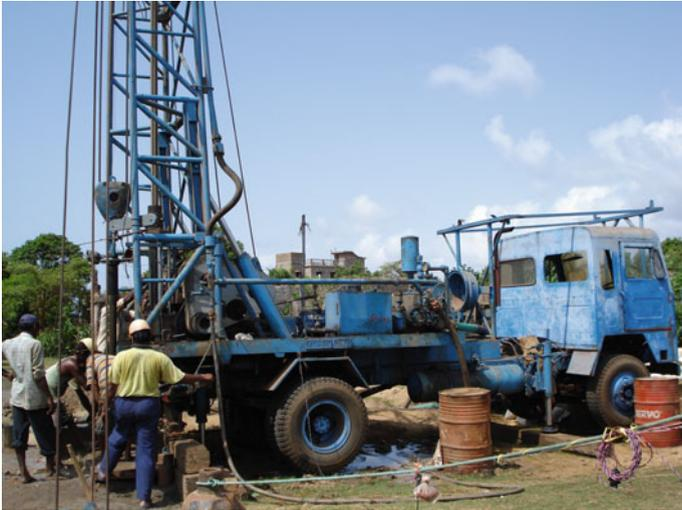
**Fig. 4.7** Drilling to tap water from the deep aquifer at Chakradharpur
