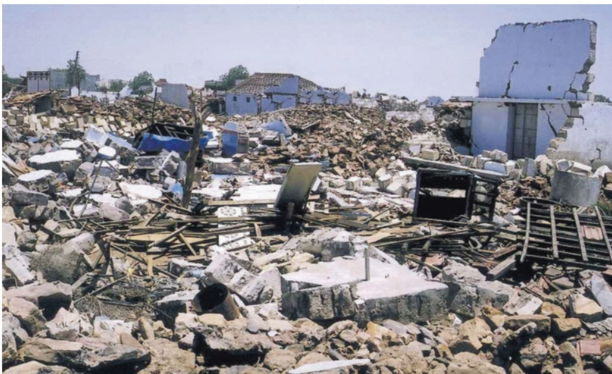
Fig. 1.4 Damage during 2001 Bhuj earthquake
