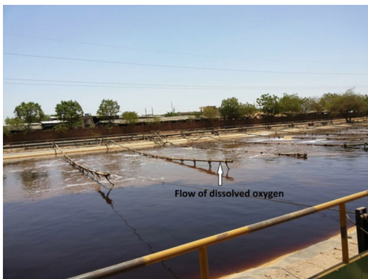
Fig. 10.3 Aeration tank showing flow of dissolved oxygen
