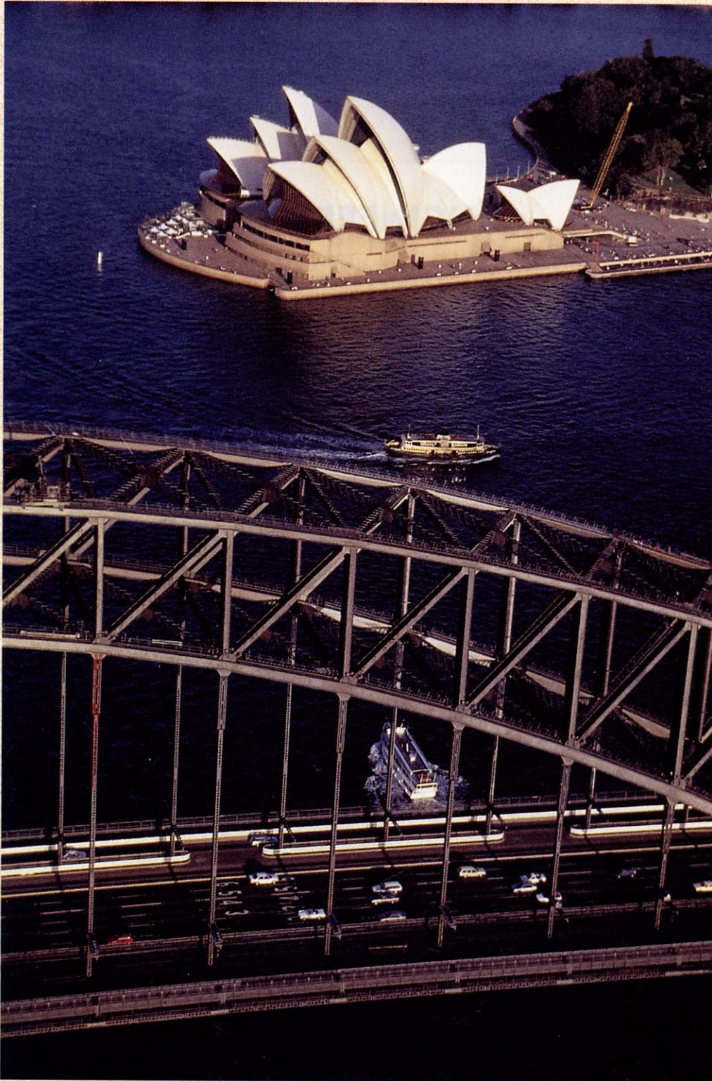
Structures which support large forces must be designed with the principles of mechanics foremost in mind. In this view of Sydney Harbor, one can see several examples of such structures.
