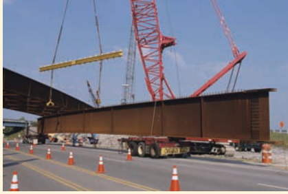
Bridge girder with overhang during transport to the construction site
