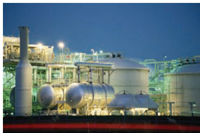
Cylindrical storage tanks in a petrochemical plant
