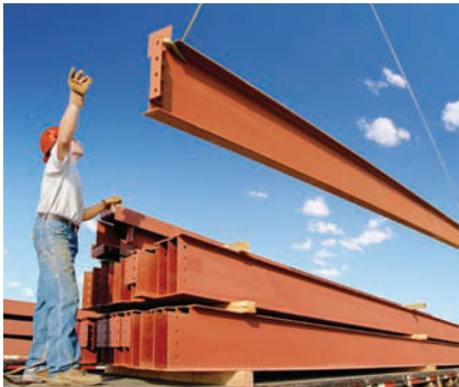
Bending due to self weight of beam and axial compression due to horizontal component of cable lifting force
