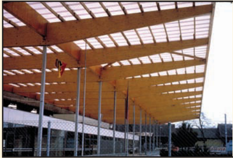
Cantilever portion of roof structure
