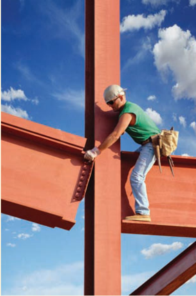
Slender steel column with lateral support near mid-height
