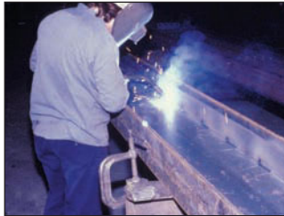
FIG. 5-17 Welder fabricating a large wide flange steel beam (Courtesy of AISC)
