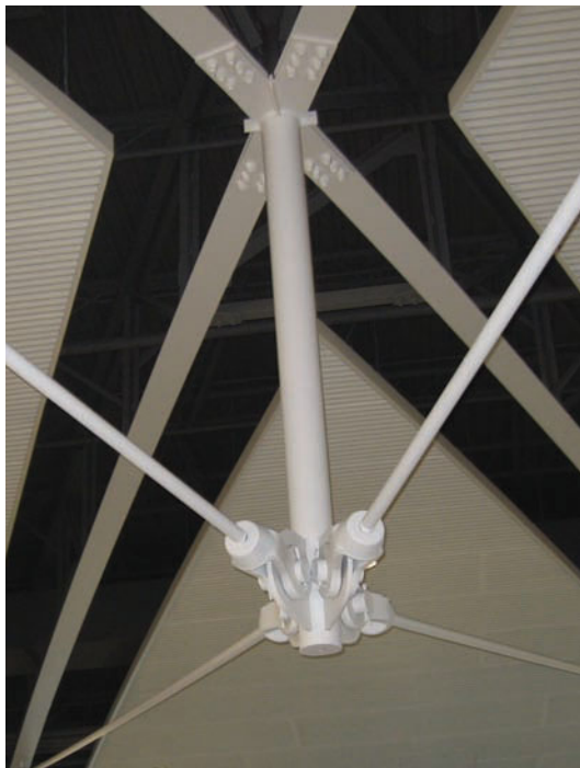
Cable and strut at typical joint of airport concourse roof
