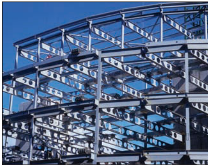
Nonprismatic beams with cutouts in their webs
